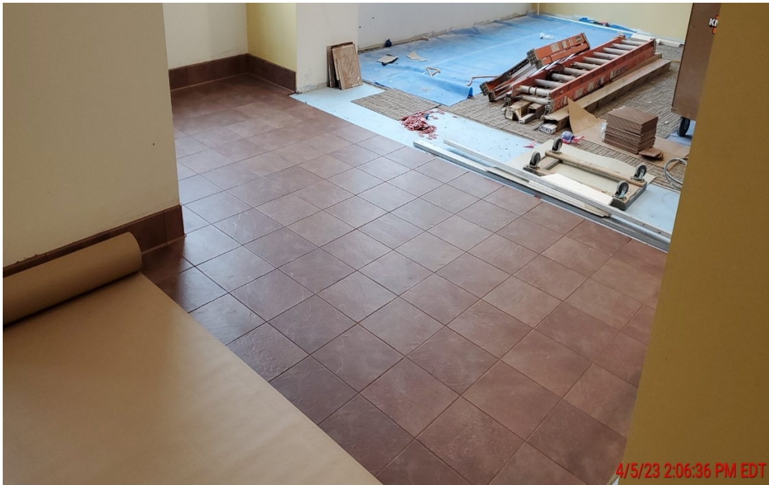
Photo #6 –Flooring in Progress (4/5/23)
