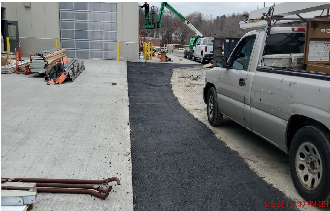
Photo #4 – Exterior Concrete Pads Placed (4/5/23)
