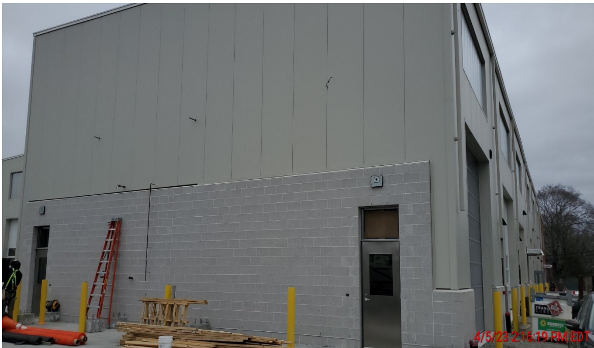
Photo #10 – PEMB Wash Bay Exterior (4/5/23)
