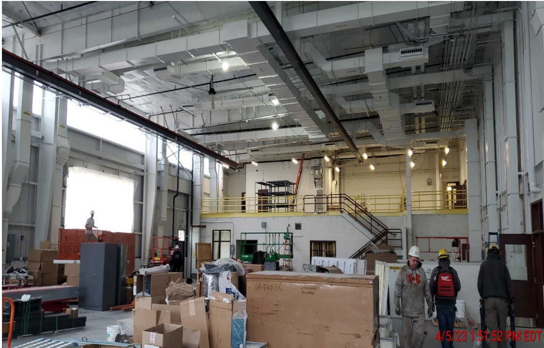
Photo #5 –PEMB Maintenance in Progress (4/5/23)
