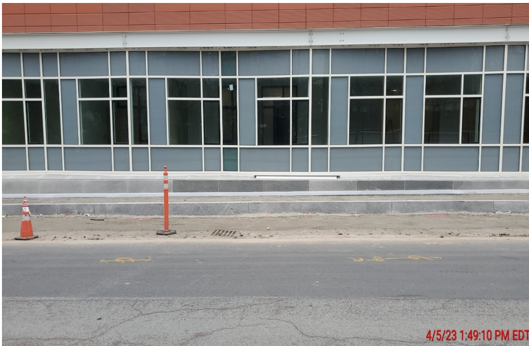
Photo #2 – Building E Curbing and Sidewalk in Progress (4/5/23)
