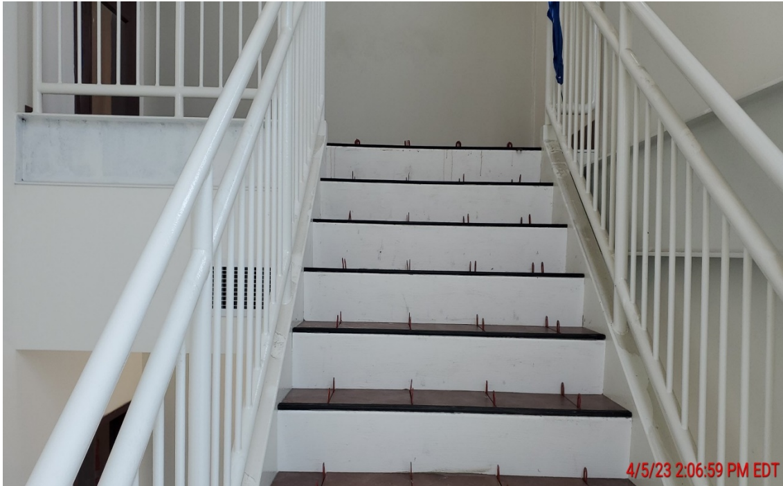
Photo #7 – Stairs and Railings in Progress (4/5/23)
