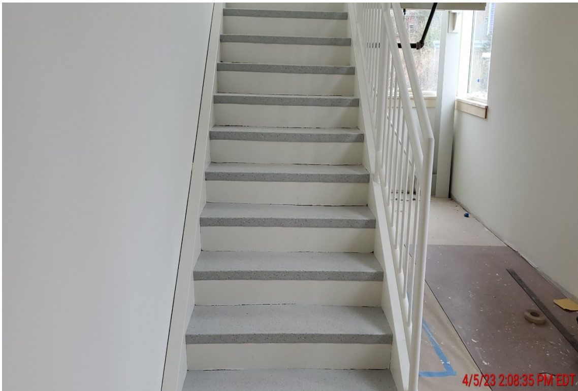
Photo #8 – Stairs and Railings in Progress (4/5/23)
