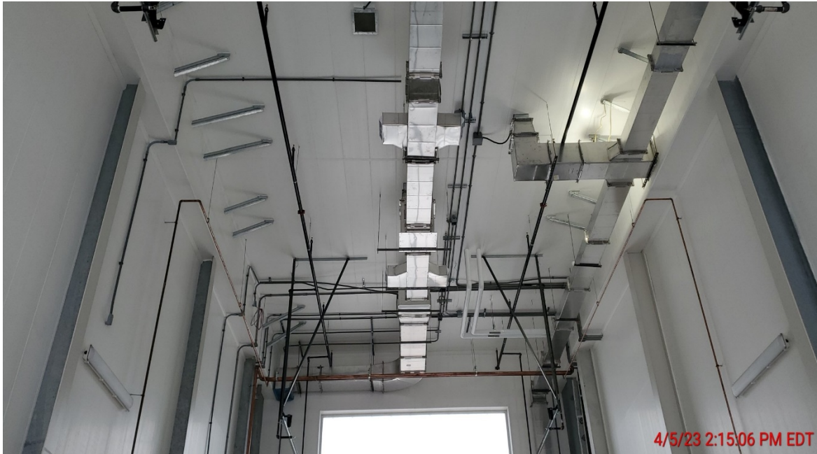
Photo #9 – Wash Bay MEPFP in Progress (4/5/23)
