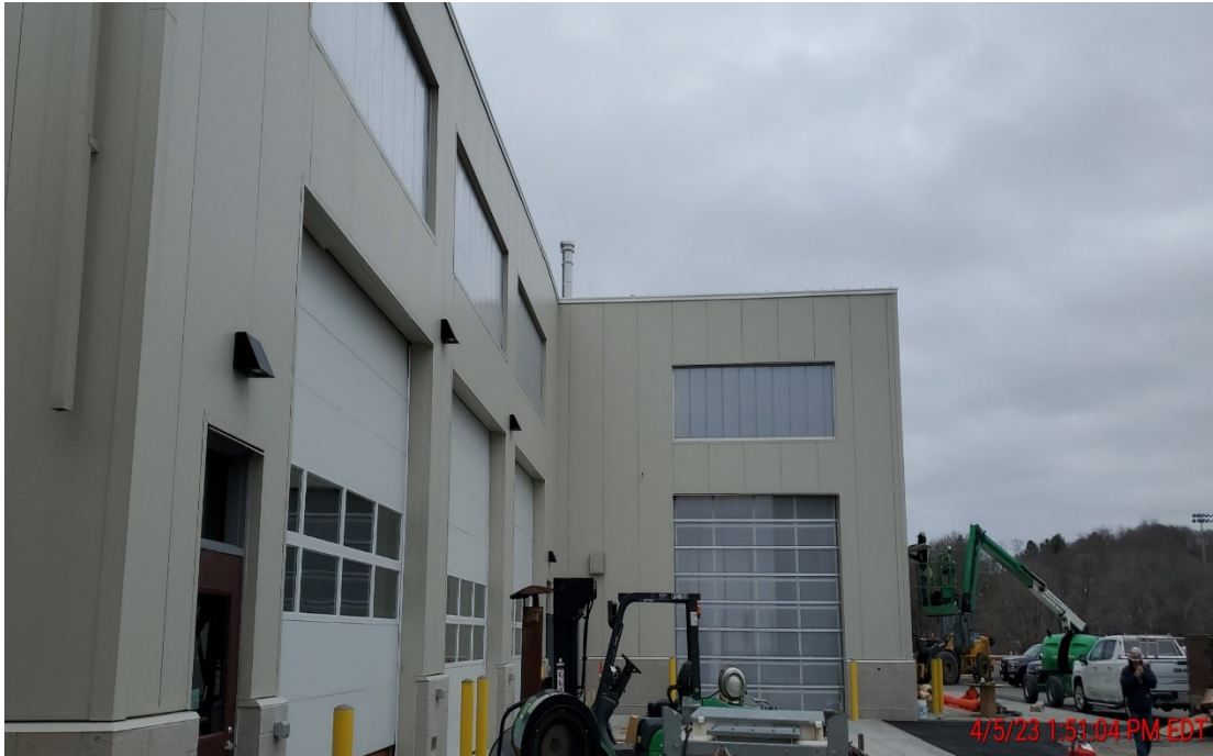
Photo #3 – PEMB Exterior in Progress (4/5/23)
