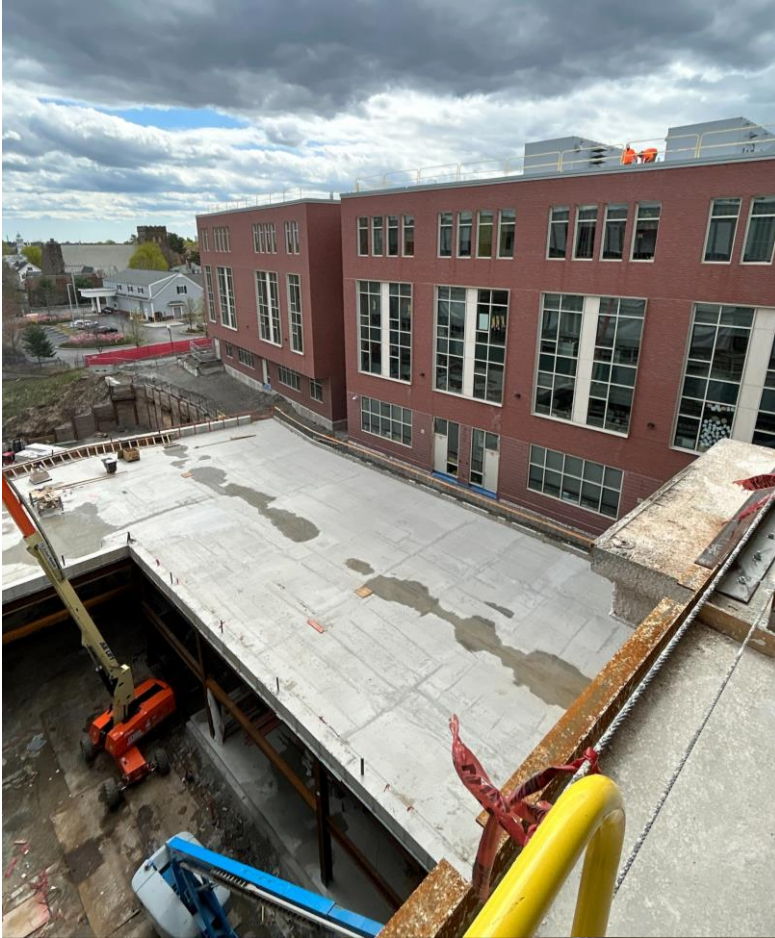
Plaza with Courtyard below
