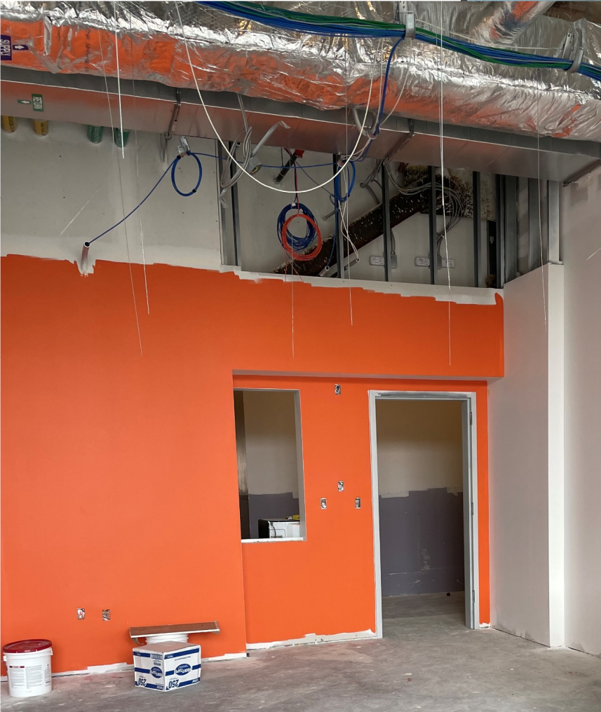
Drywall taping and sanding complete and painting progressing
