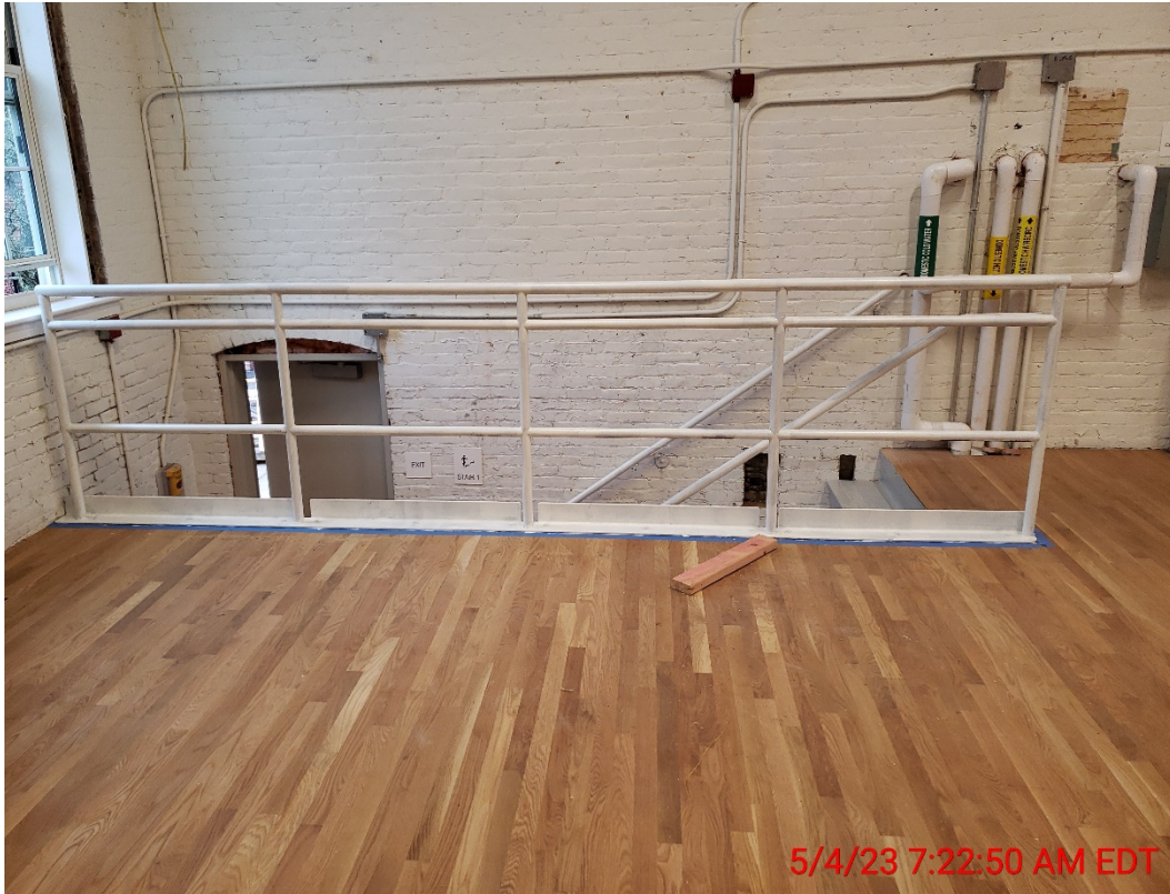
Photo #7 – Building A Facilities Work Shop Mezzanine (5/4/23)
