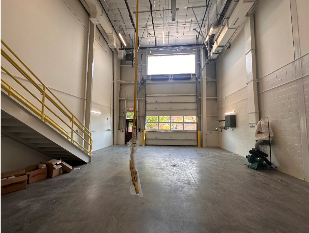
Photo #1 – Building E Maintenance Bay - Typical (05/12/23)
