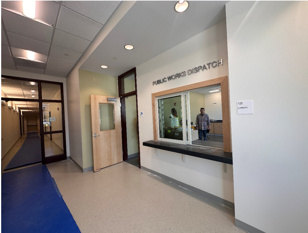
Photo #5 – Building E Admin – Dispatch (5/12/23)
