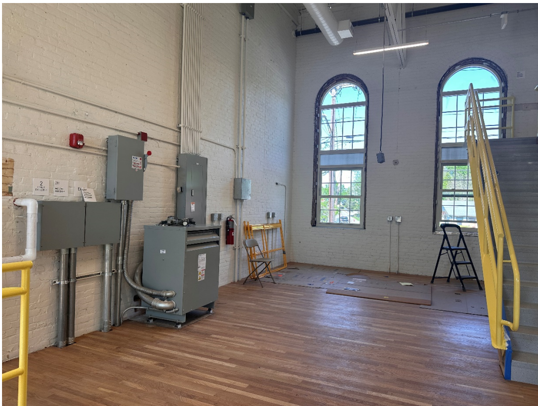
Photo #6 – Building A Facilities Work Shop Level 1 (5/12/23)
