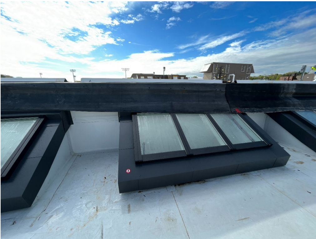
Photo #4 – Building E Admin. Skylights Installed (5/3/23)
