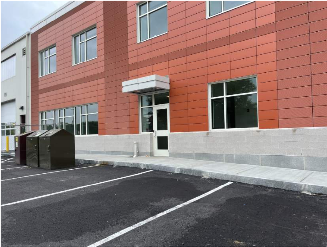
Photo #7 – Building E Administration Side Entrance (6/12/23)
