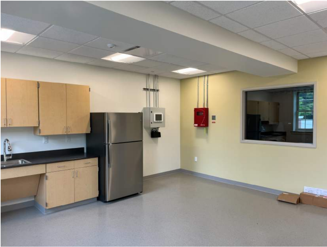
Photo #1 – Building A Conference/Break Room (6/9/23)
