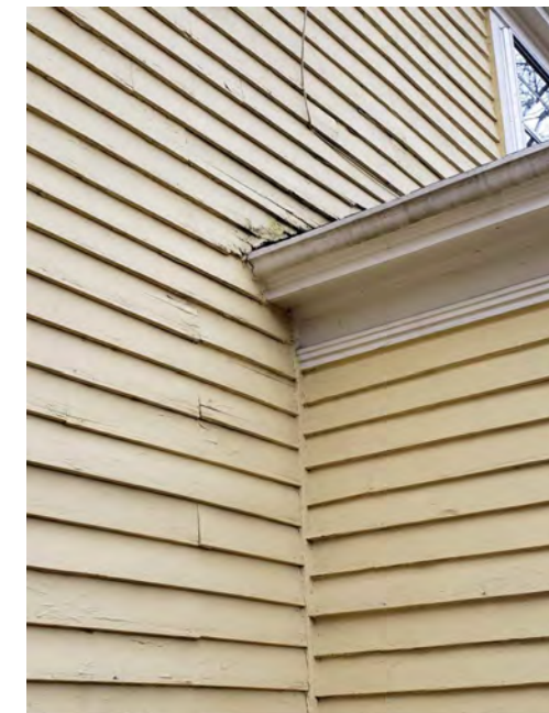
REMOVE & REPLACE SIDING
