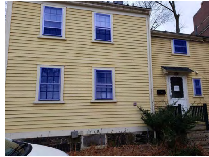
REMOVE STORM WINDOWS AND SEALANT, TYP.
