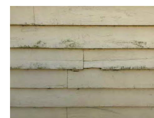
REMOVE, REPLACE, PRIME & PAINT SIDING 4-1/8"x46-1/2", 4-1/8"x46-3/4"
