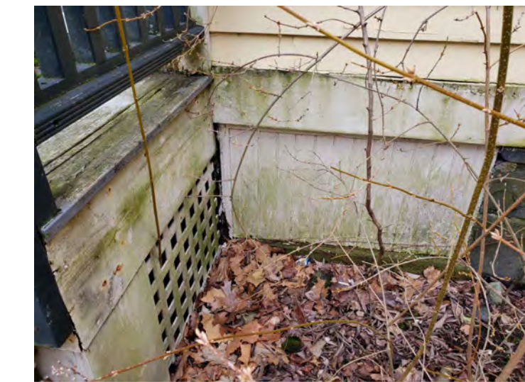
REMOVE BOARDED OVER WINDOW AND INSTALL 6" CMU.
