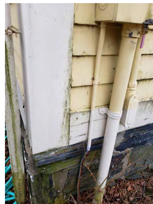
REMOVE & REPLACE SPLIT END BOARD
