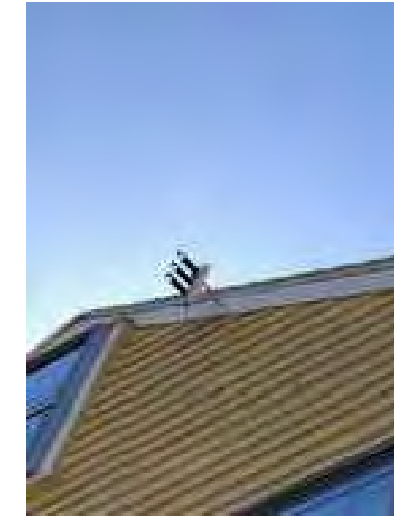
REMOVE ELECTRICAL FITTING
