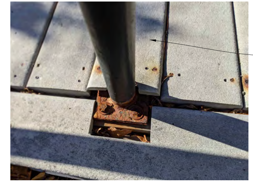
RAMP POST PHOTO "A"
