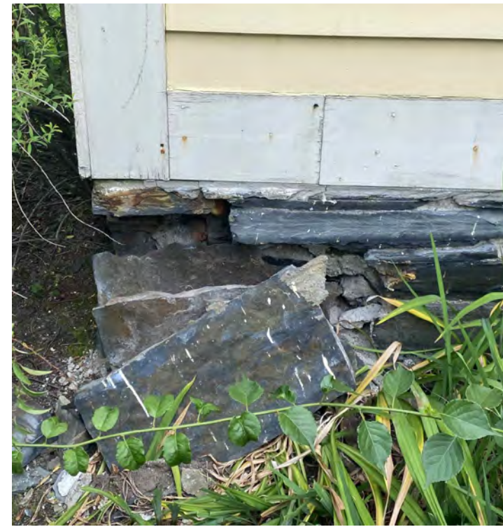
RESET AND MORTAR STONE FOUNDATION
