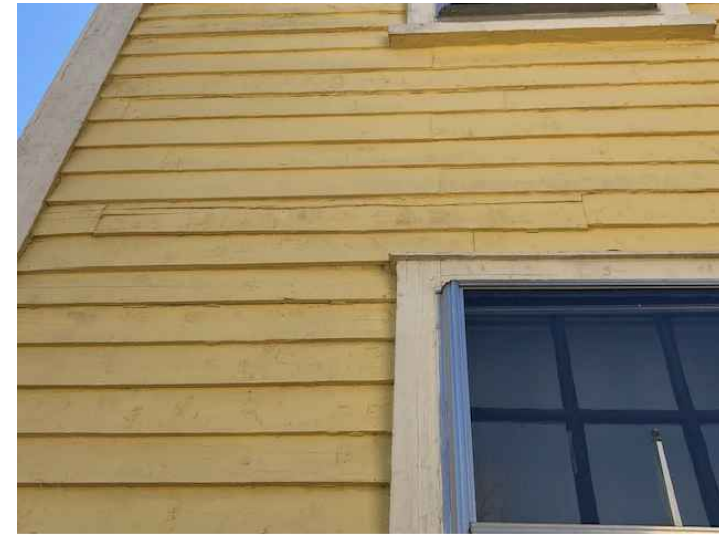
REMOVE & REPLACE SIDING 4-1/4"x48-1/2"
