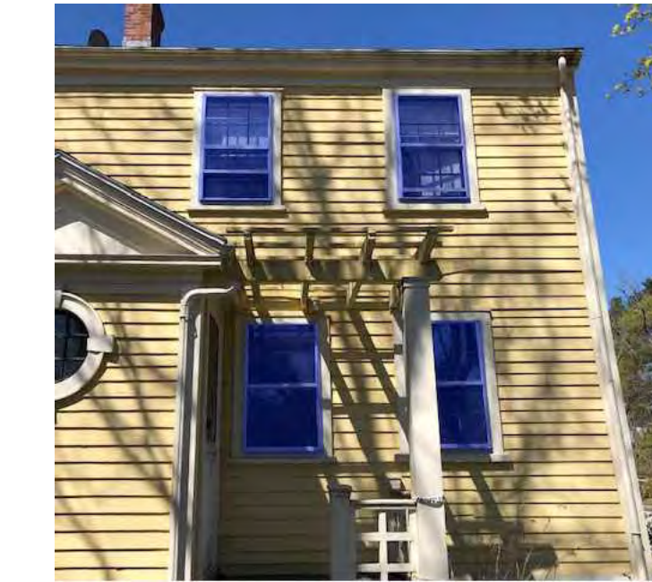
REMOVE STORM WINDOWS AND SEALANT - TYP.
