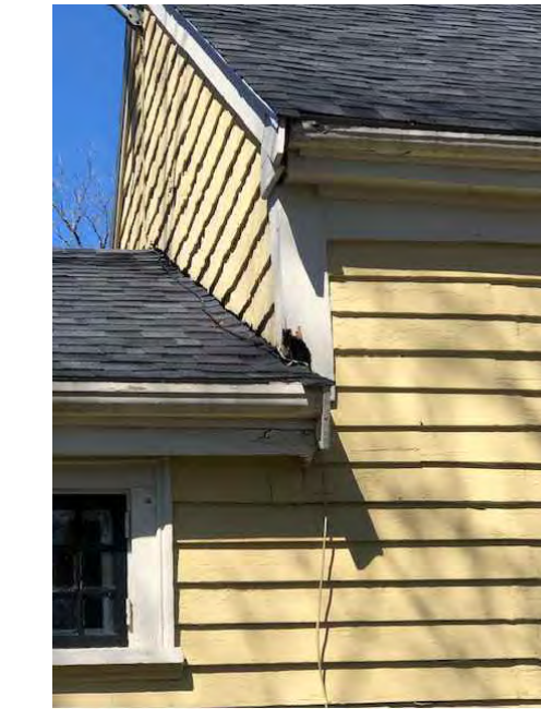
REMOVE & REPLACE CORNERBOARD THAT IS PULLING AWAY FROM ROOF
