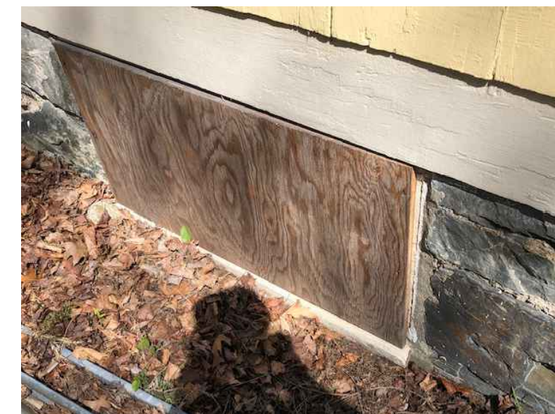
REMOVE & REPLACE BASEMENT WINDOW
