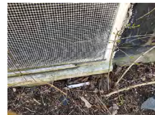
REMOVE & REPLACE BASEMENT WINDOW
