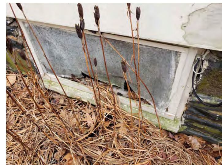
REMOVE & REPLACE BASEMENT WINDOW
