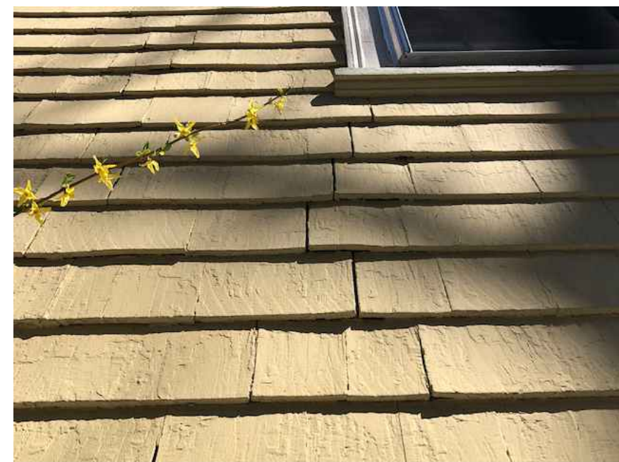
NAIL LIFTING SHINGLES DOWN AND PAINT AS NECESSARY
