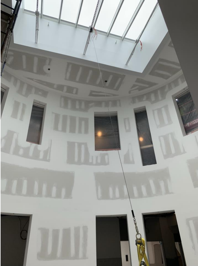
Photograph 4: Progress of lightwell
