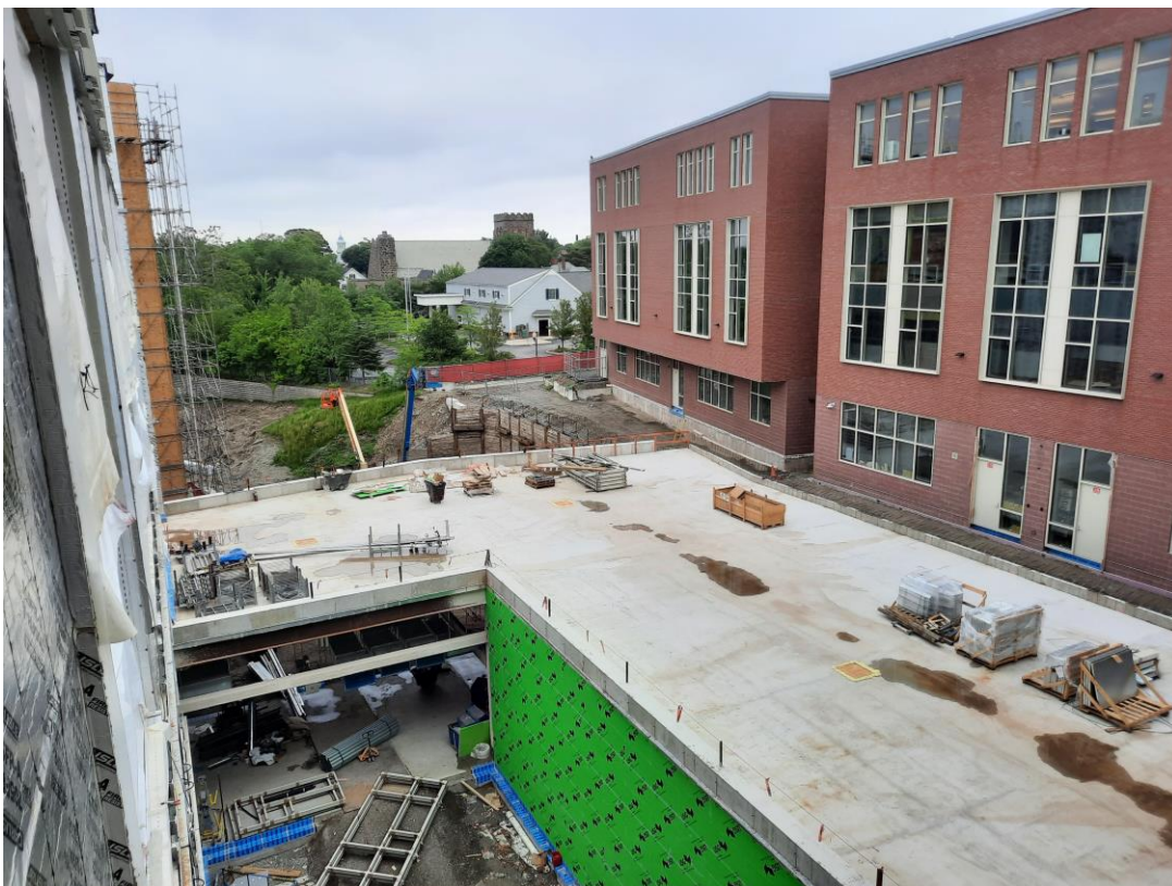
Photograph 3: Looking South onto plaza from 4 th Floor connecting corridor
