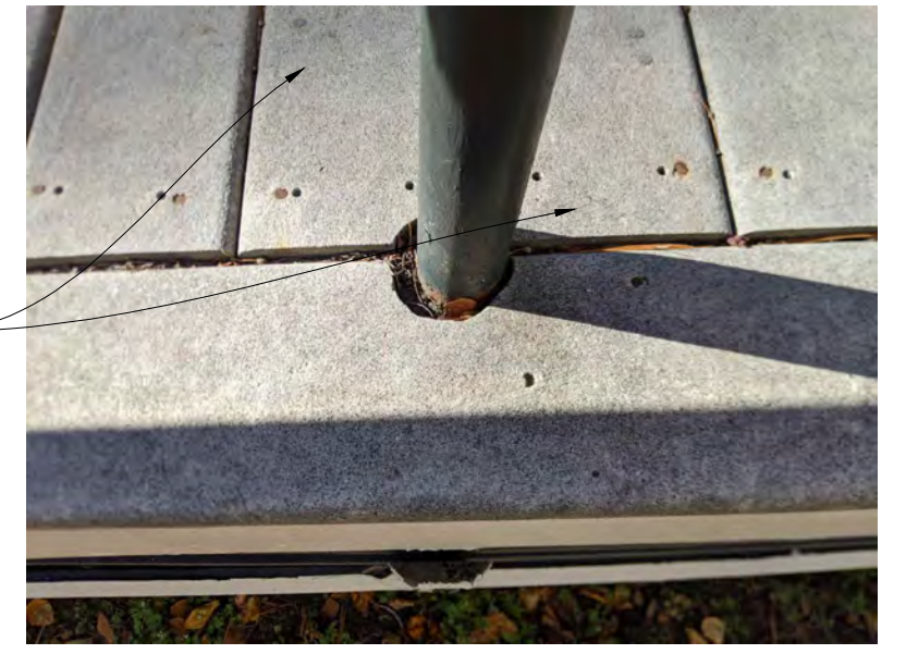
RAMP POST PHOTO "B"
