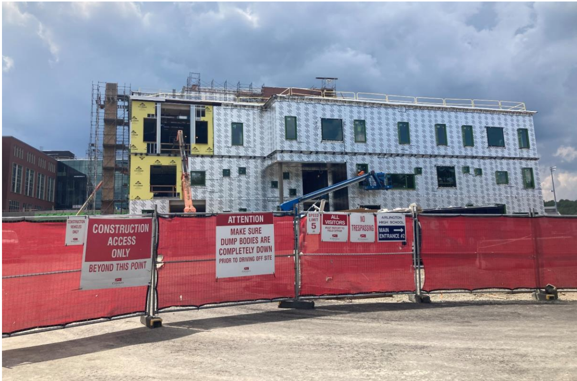
Photograph 1: Phase 2 East Elevation (Mill Brook Dr)
