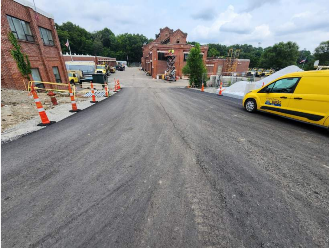
Photo #5 – Binder Placed at Lower Portion of the Site (7/18/23)
