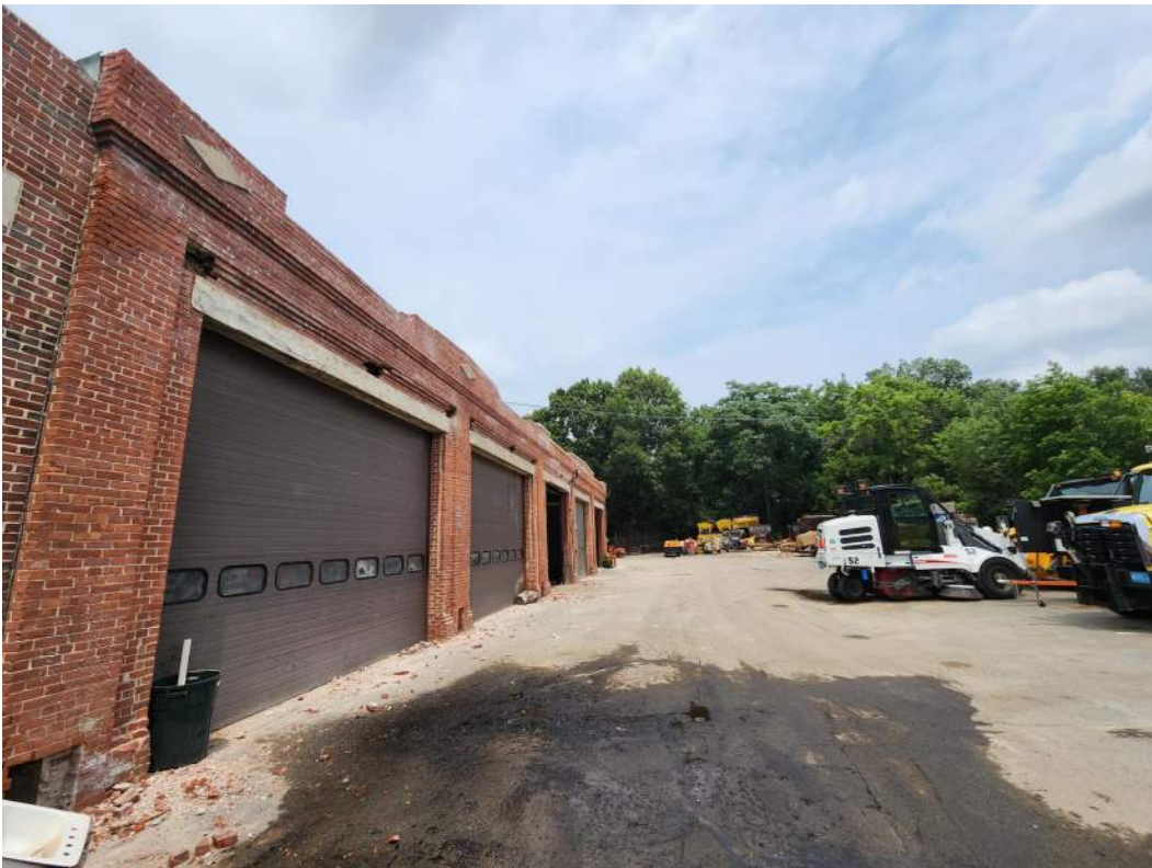
Photo #4 – Masonry Rebuilding/Repointing at Building D (7/18/23)
