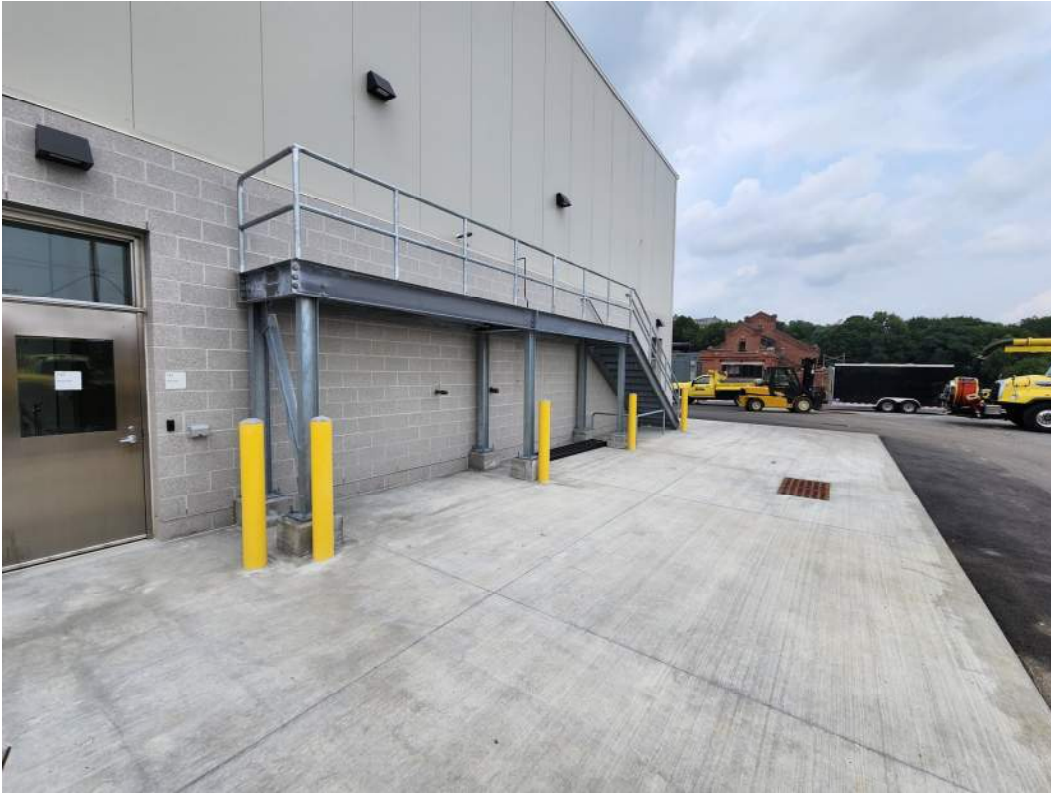
Photo #1 – Washbay Knockdown Pad Stair and Railings (7/18/23)
