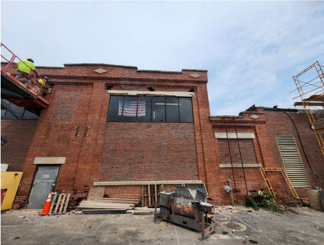
Photo #3 – Masonry Repointing/Rebuilding at Building D (7/18/23)
