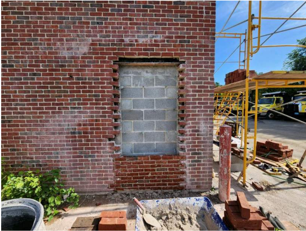
Photo #5 – Building D Masonry Infill in Progress (8/22/23)
