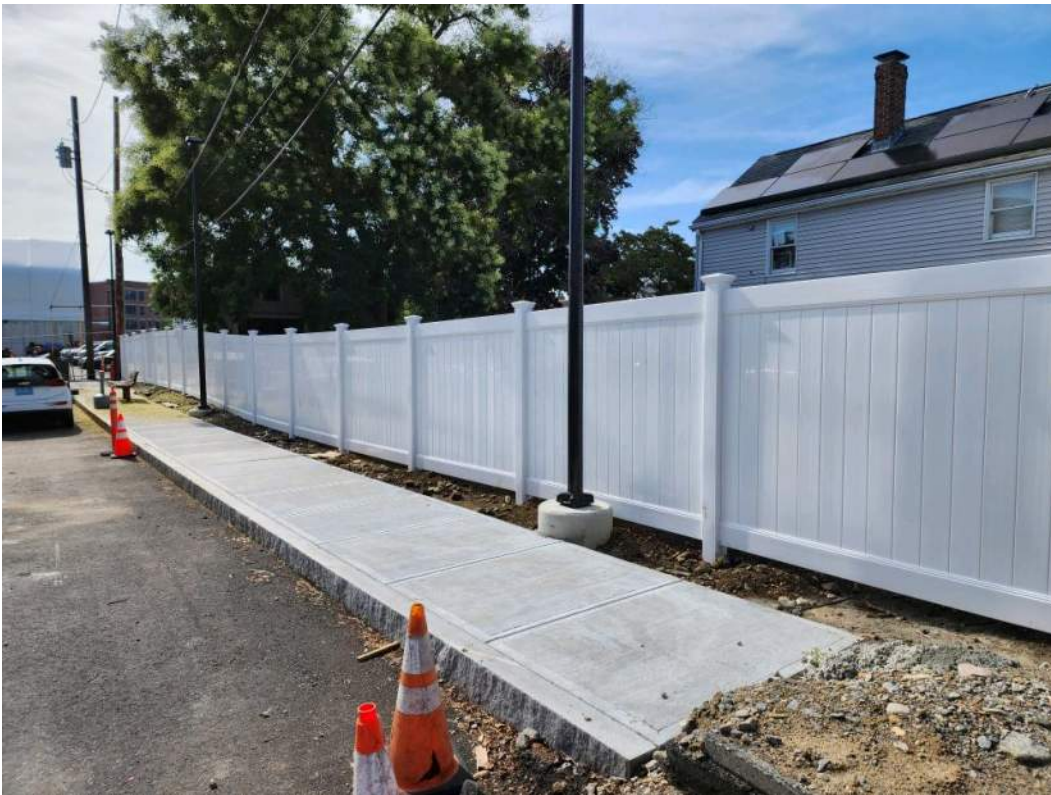
Photo #8 – Fence Install (8/22/23)
