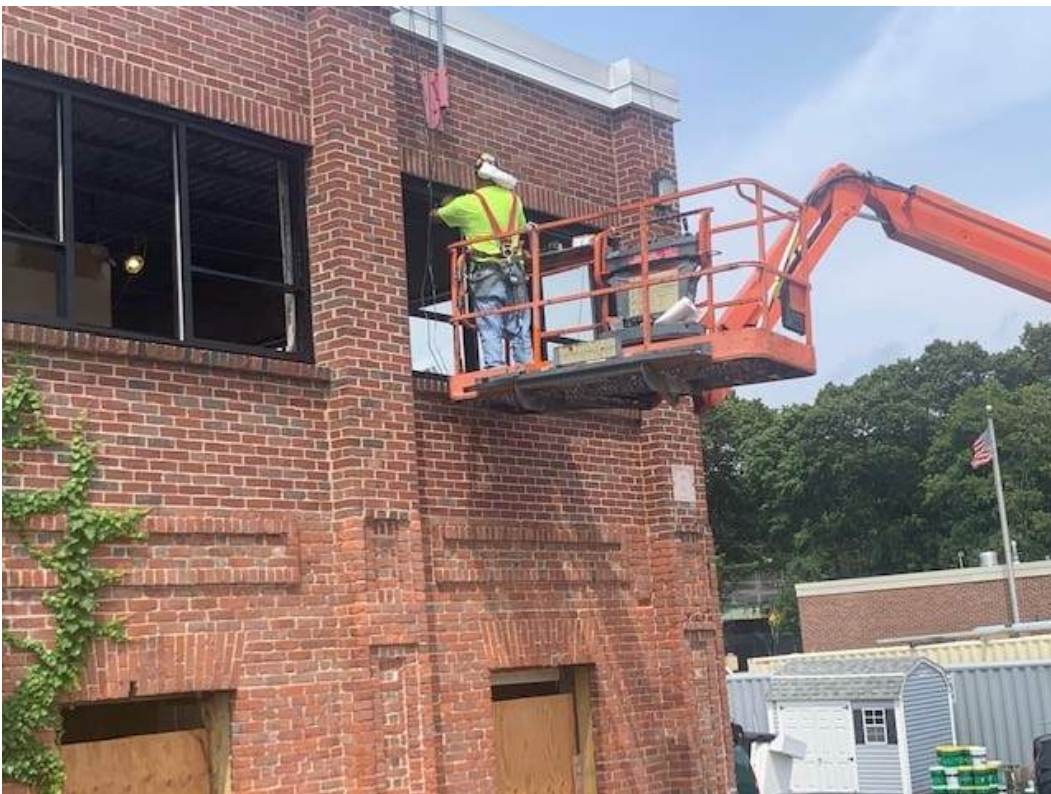
Photo #4 – Building B Masonry in Progress (8/10/23)
