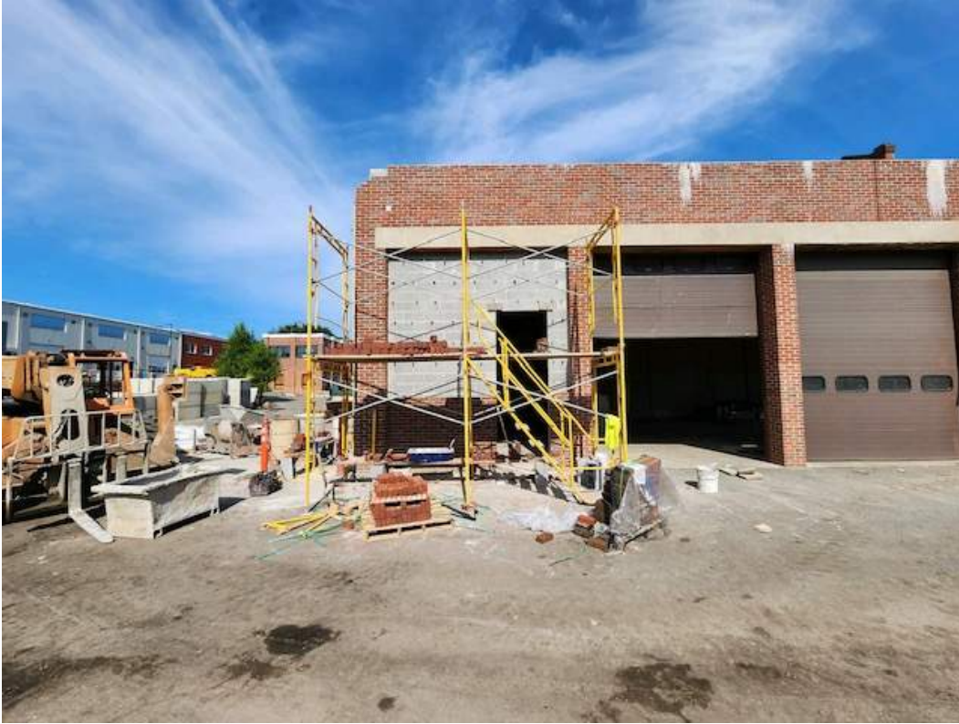
Photo #7 – Building D Masonry Infill in Progress (8/22/23)
