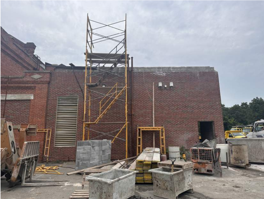
Photo #1 – Building D Masonry in Progress (8/10/23)
