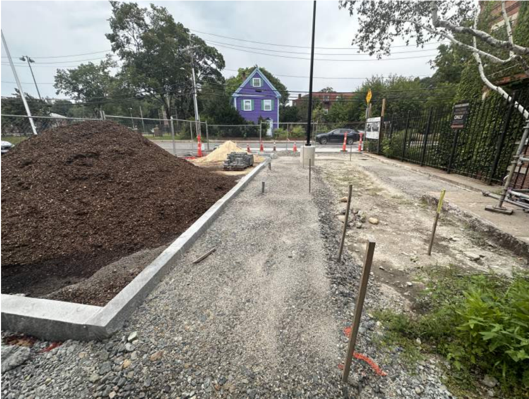
Photo #3 – Building B Curb Install in Progress (8/10/23)
