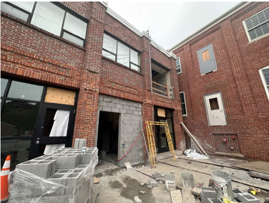
Photo #2 – Building B CMU Infill in Progress (8/10/23)
