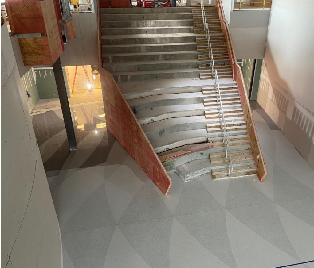
Photograph 1: Forum Stair Terrazzo Floor Progress
