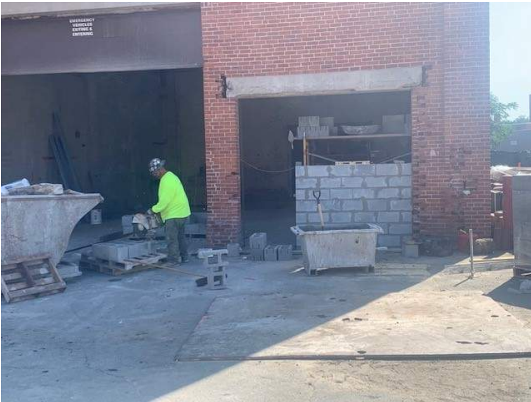
Photo #8 – Building D CMU in Progress (9/21/23)
