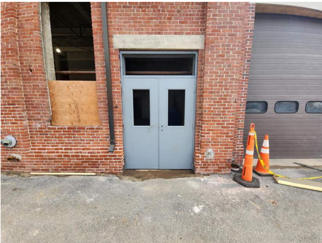
Photo #4 – Building D New Exterior Door Installed (9/19/23)
