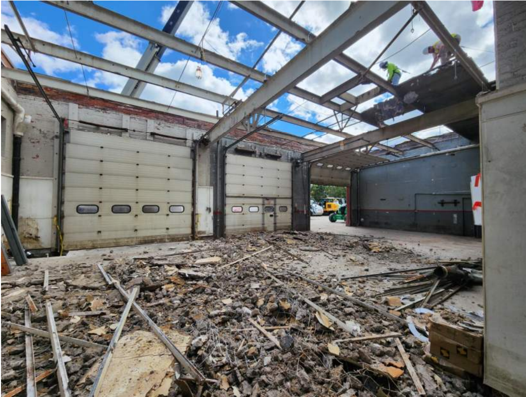
Photo #1 – Building D Roof Demo in Progress (9/19/23)
