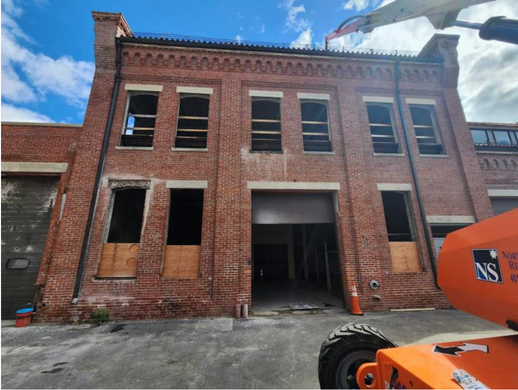
Photo #5 – Building D Window Demo in Progress (9/19/23)
