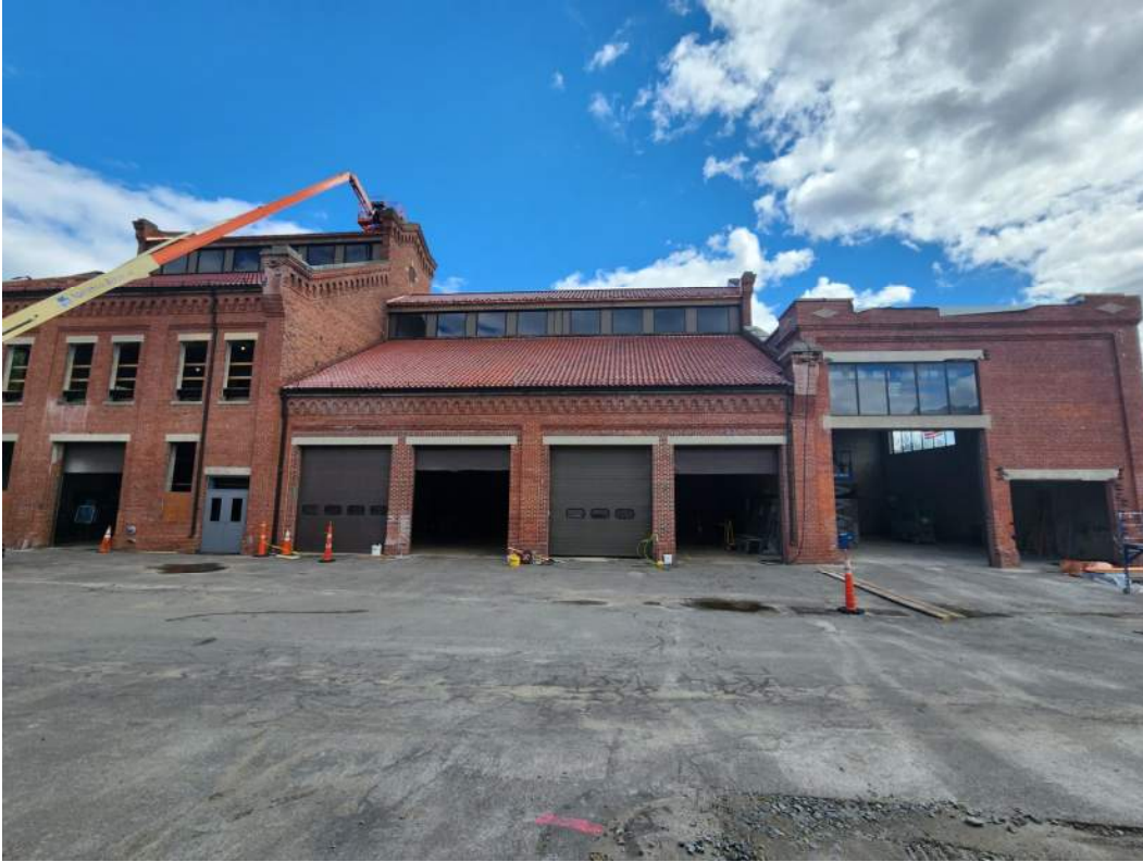
Photo #7 – Building D Terracotta Roof in Progress (9/19/23)
