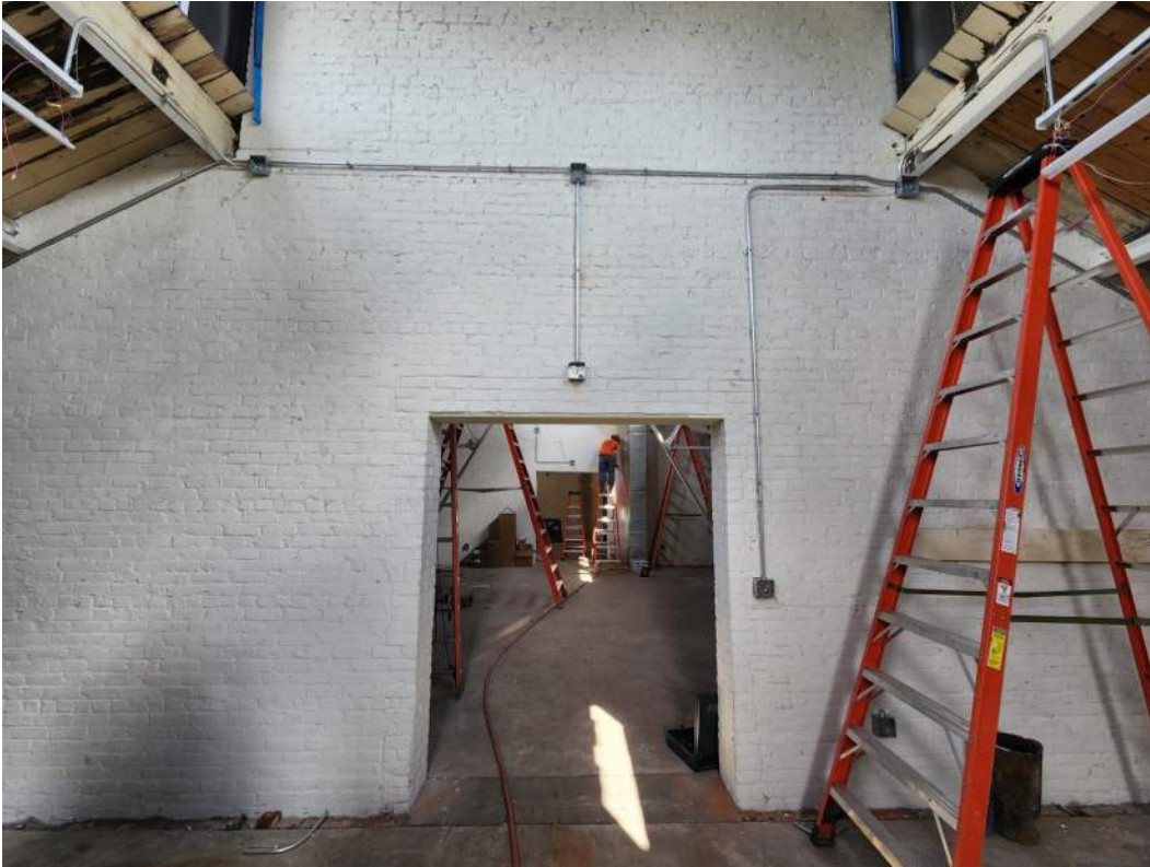
Photo #3 – Building D 2 nd Floor MEP in Progress (9/19/23)
