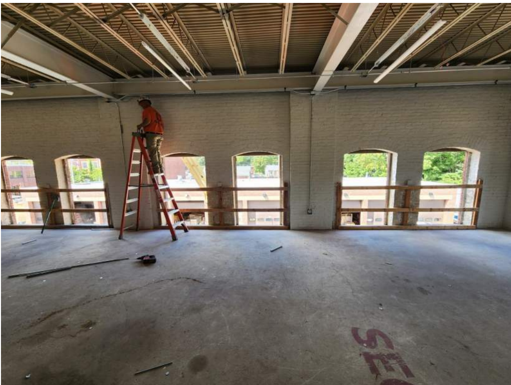
Photo #2 – Building D Window Demo in Progress (9/19/23)
