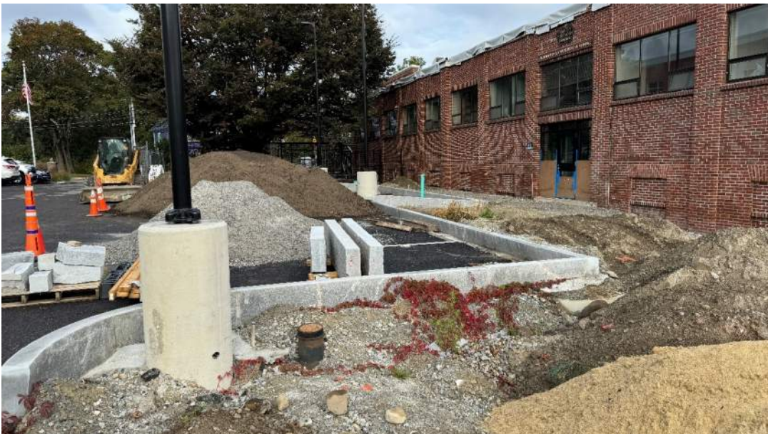
Photo #4 – Sitework in Progress (10/10/23)
