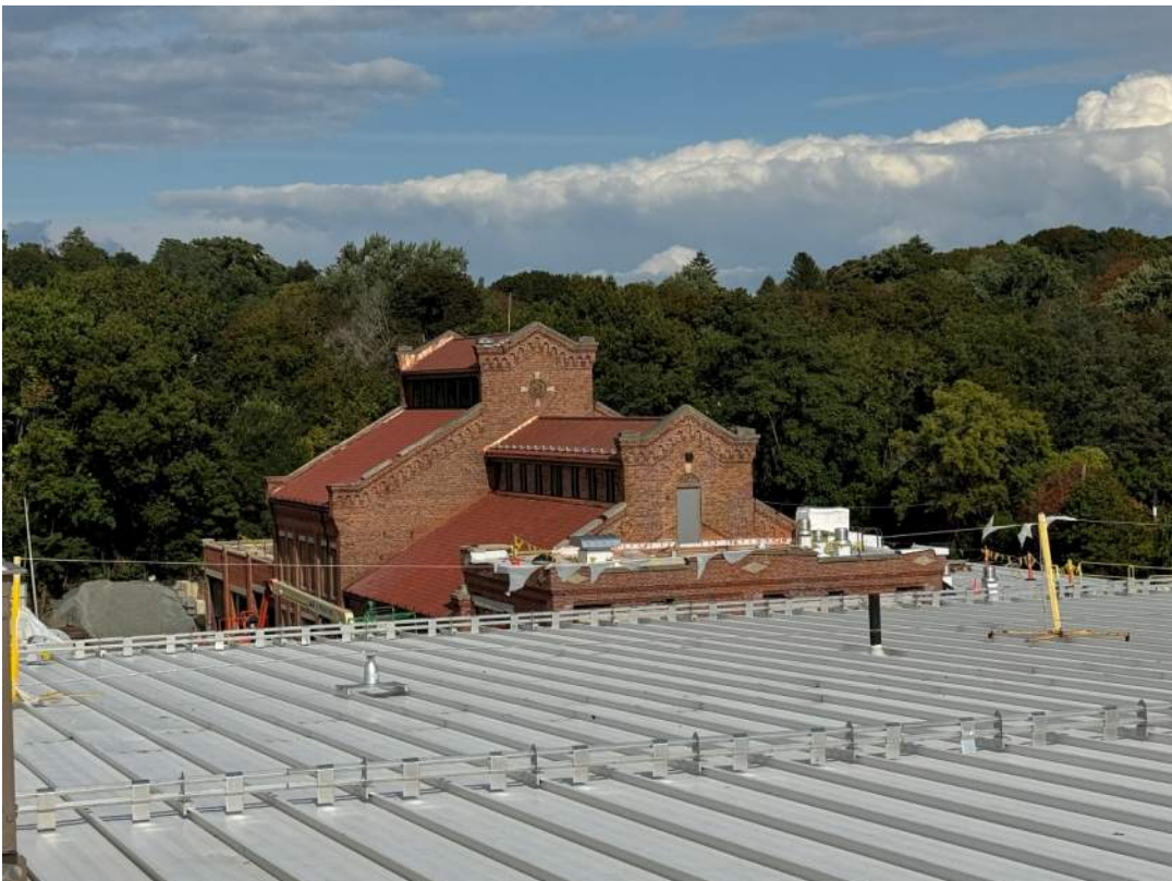
Photo #6 – Building E Roof and Wall Panels Complete (10/10/23)
