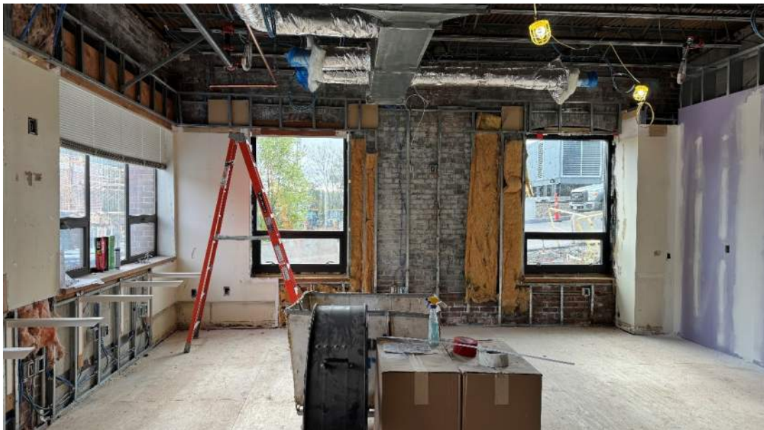
Photo #2 – Building B MEP in Progress (10/10/23)
