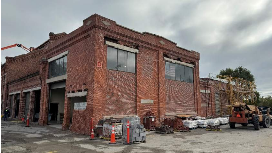
Photo #7 – Building D Lintel Replacement (10/17/23)
