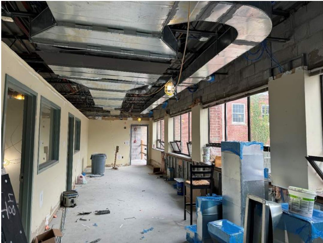
Photo #1 – Building B MEP in Progress (10/10/23)
