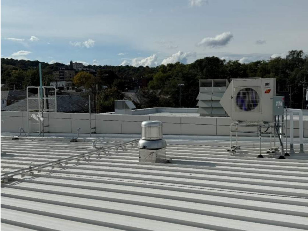
Photo #5 – Building E Roof and Wall Panels Complete (10/10/23)
