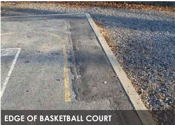
COURT CRACKING AND PAINT CHIPPING
