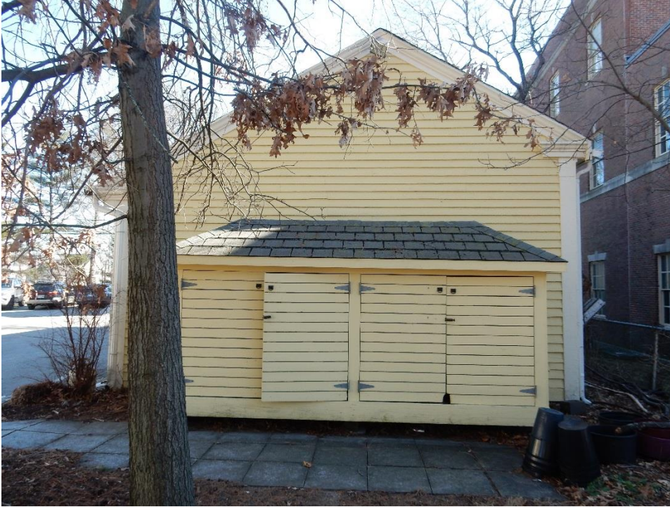
3. West face of Whittemore Robbins Carriage House. Detached shed in foreground.
