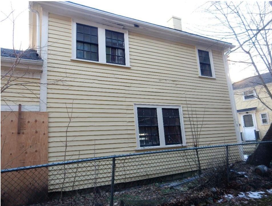
4. East end of South face of Whittemore Robbins Carriage House
