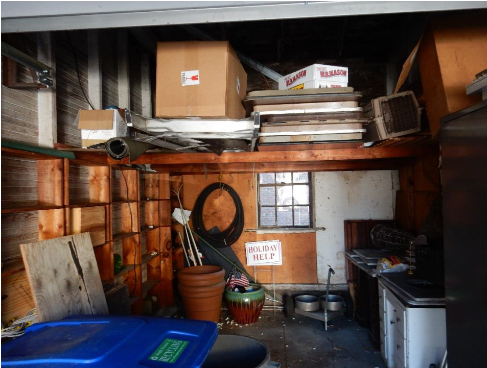
14. West most bay in one-story portion. Area is dry. A makeshift loft supports storage.
