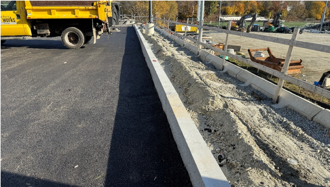
Photo #4 – Curb Installation Complete and Paving (11/21/23)
