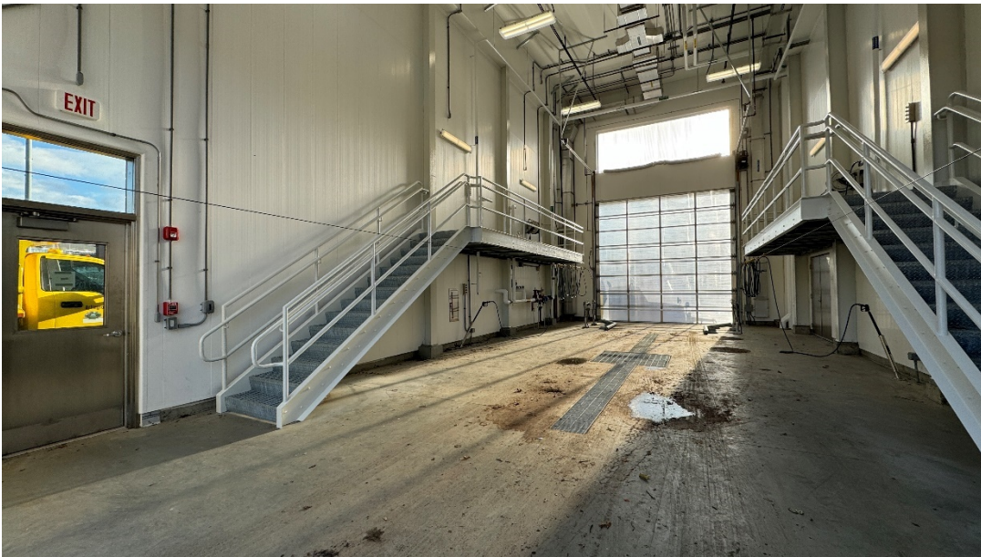
Photo #6 – Building E Stairs Complete (11/21/23)
