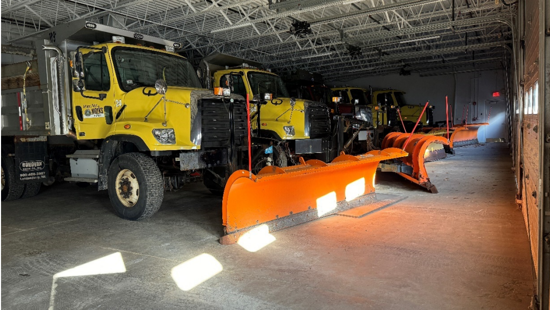
Photo #5 – Building C Clean Out Repair (11/21/23)
