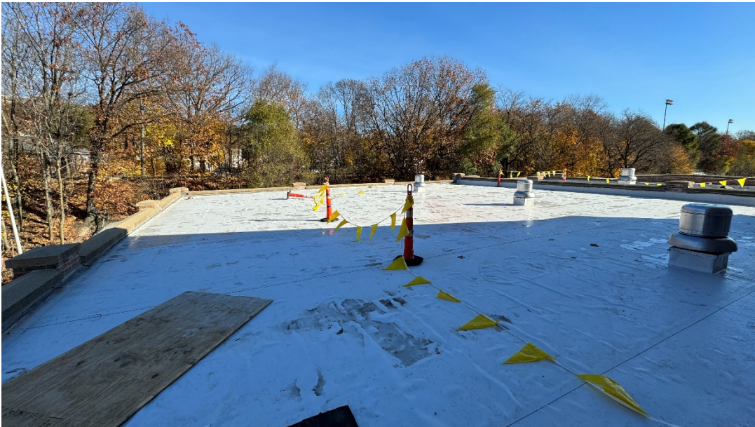
Photo #2 – Building D New Roof (11/21/23)
