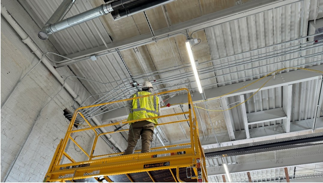
Photo #3 – Building D Electrical Work in Progress (11/21/23)
