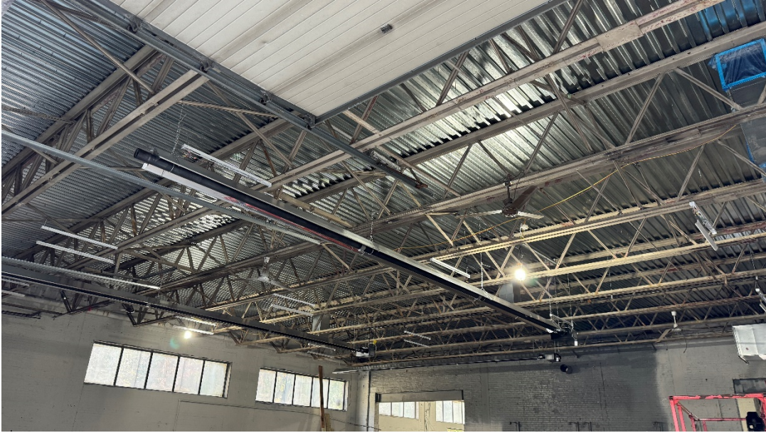
Photo #1 – Building D New Roof (11/07/23)
