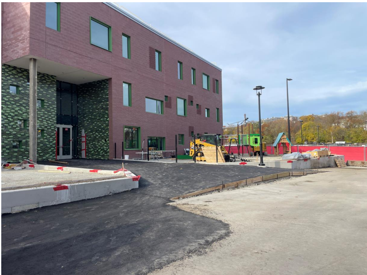
Photograph 2: East Entrance pavement progress.
