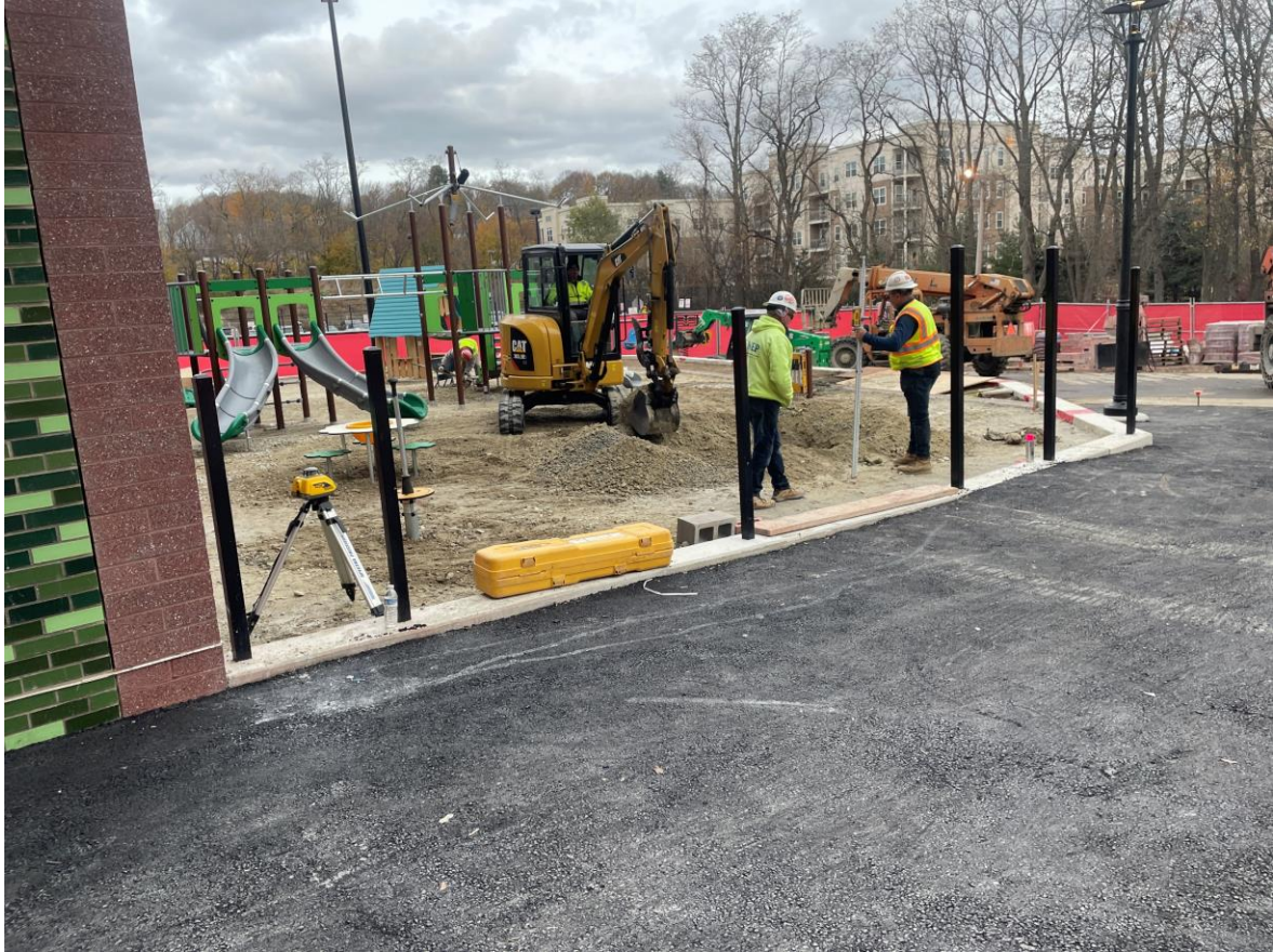
Photograph 1: Pre-School Playground fence post installation.
