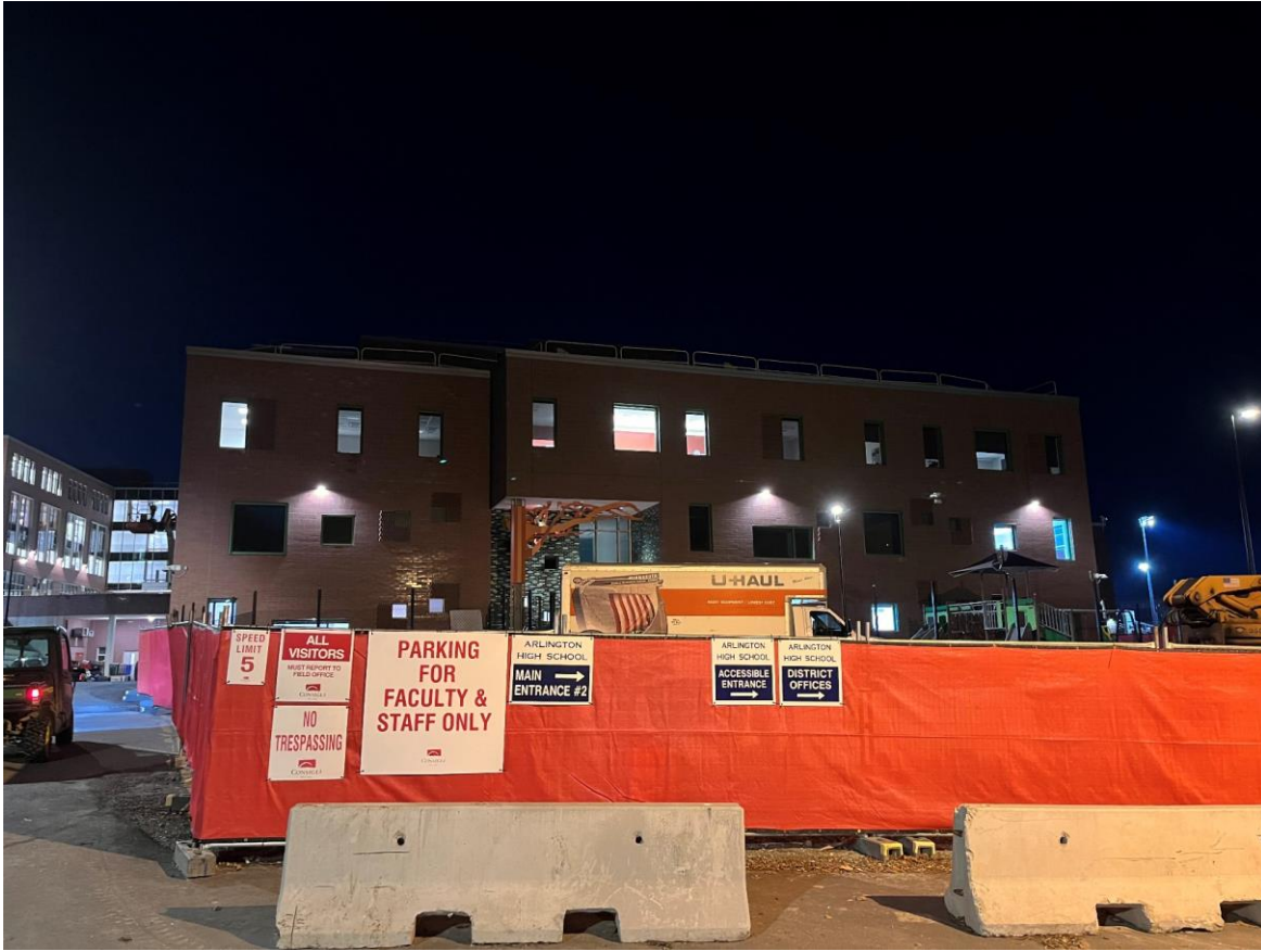
Photograph 3: East Elevation (Mill Brook Dr)
