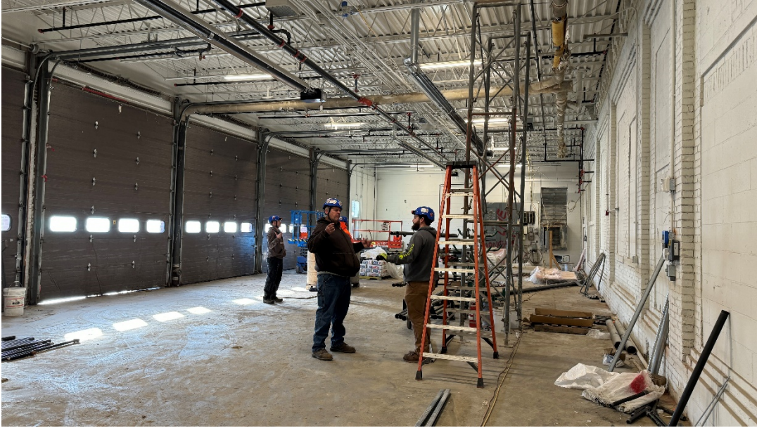
Photo #5 - Building D MEP in Progress (12/19/23)
