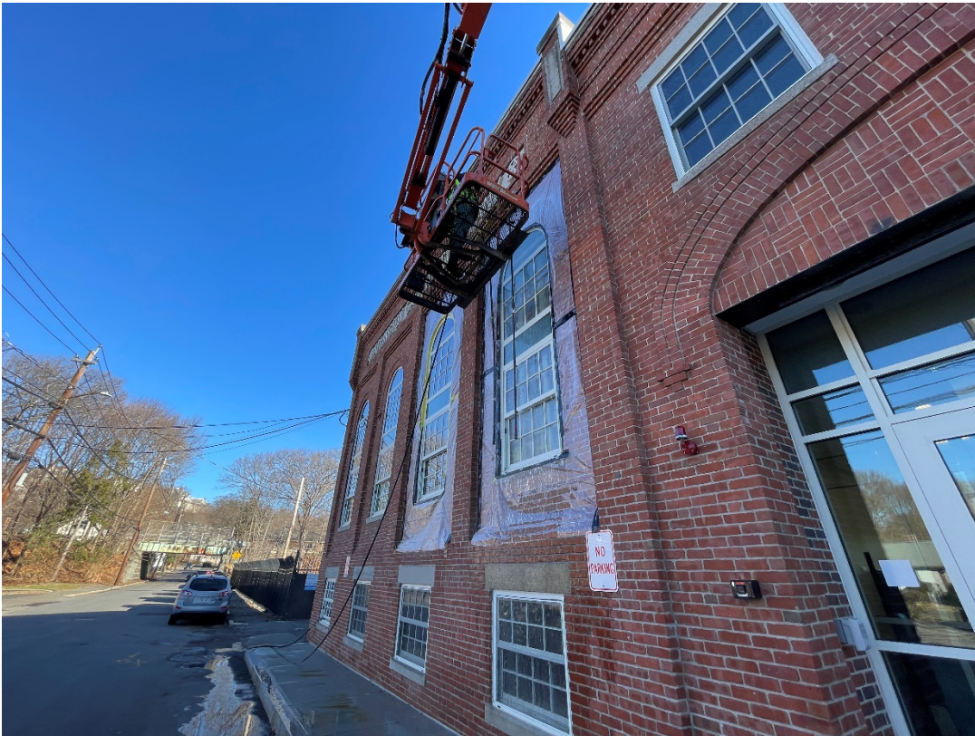
Photo #4 – Building A Window Testing - in Progress (12/19/23)
