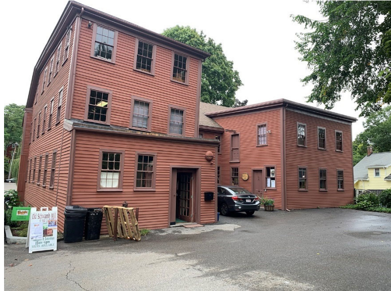
The existing Old Schwamb Mill at 17 Mill Lane [26].
