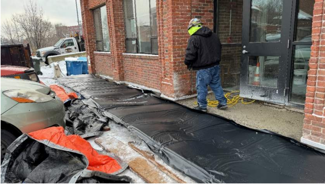
Photo #3 - Building B Sidewalk Concrete in Progress (01/09/24)
