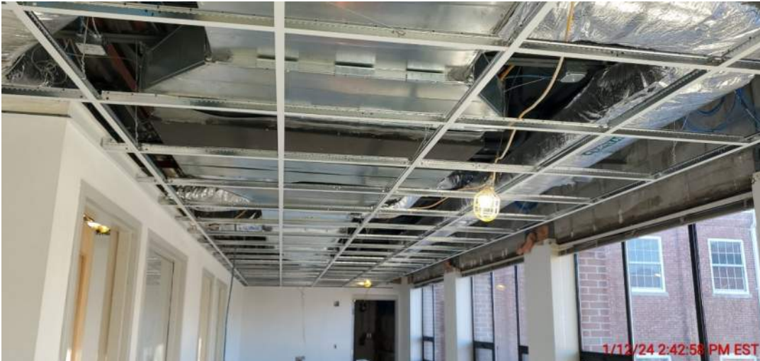
Photo #8 - Building B Ceiling Grid Layout in Progress (01/12/24)
