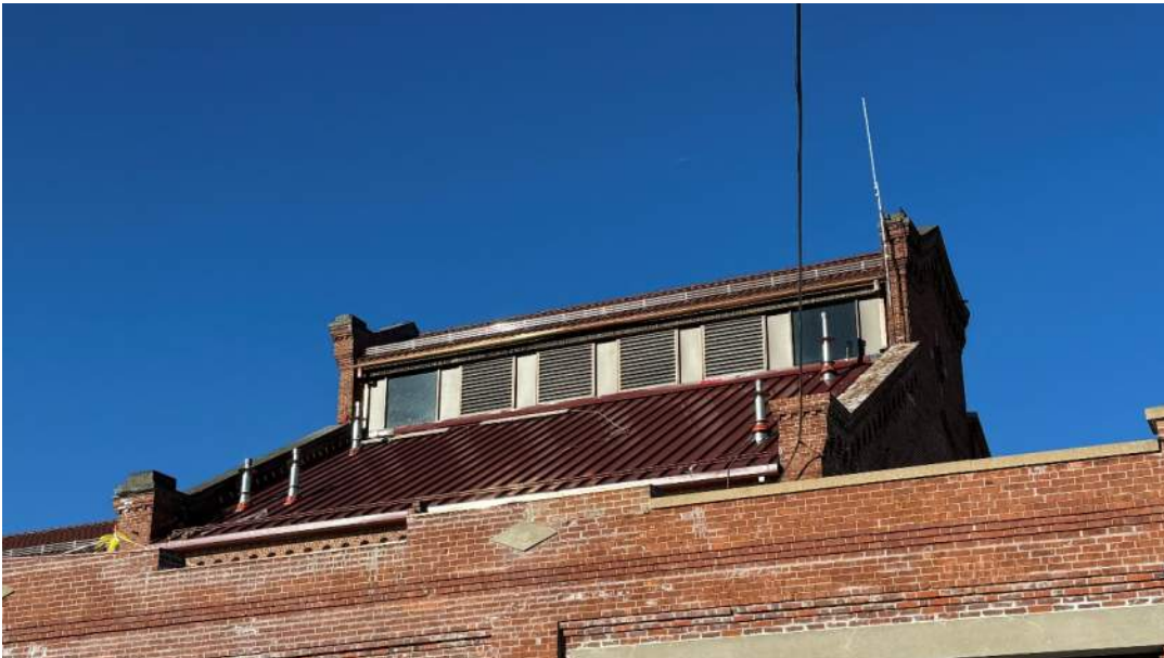
Photo #6 - Building D - New Roofs Installed (01/09/24)
