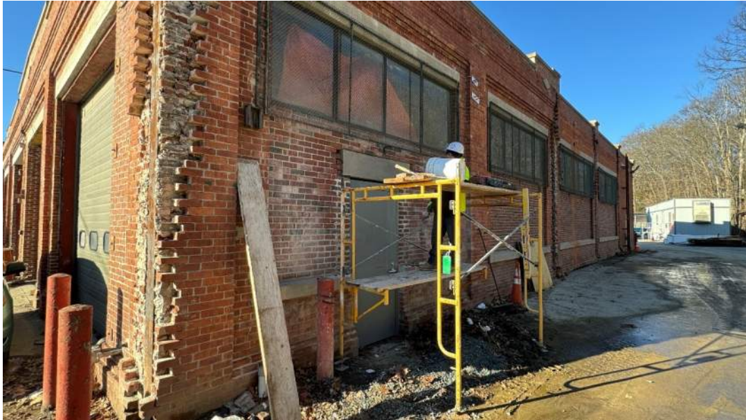
Photo #1 - Building D - Lintels Installation (01/02/24)
