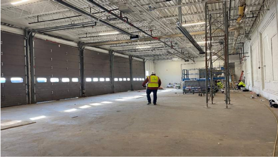
Photo #7 - Building D MEP in Progress (01/12/24)
