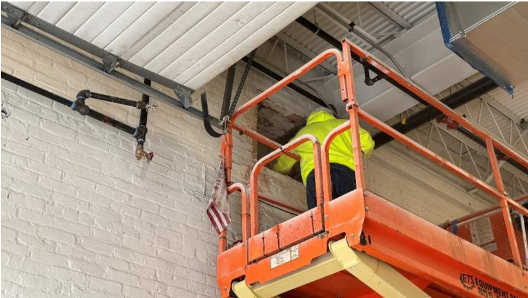
Photo #4 - Building D MEP Openings in Progress (01/09/24)
