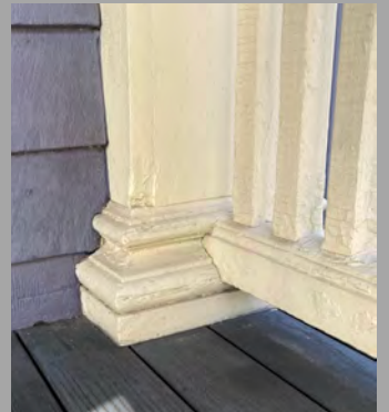
Front porch pilaster bottom
