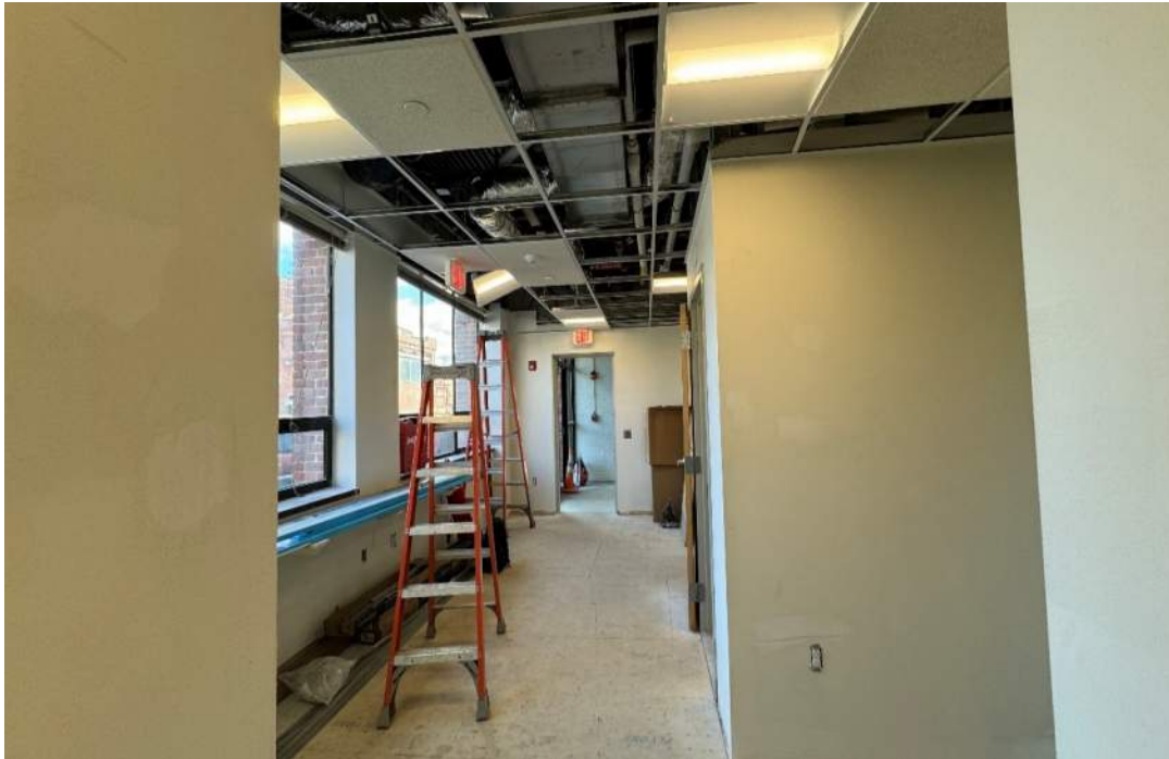
Photo #5 - Building B First Floor Interior in Progress (02/06/24)
