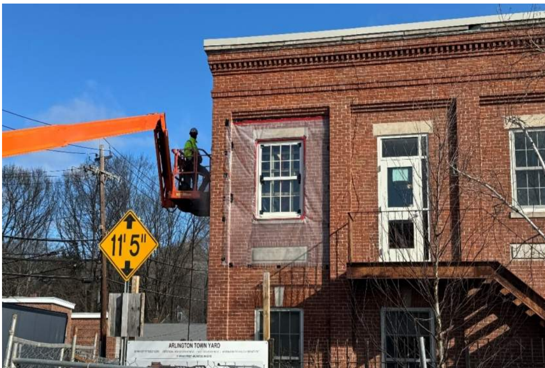
Photo #2 - Building A - Pre-Test Window (02/06/24)
