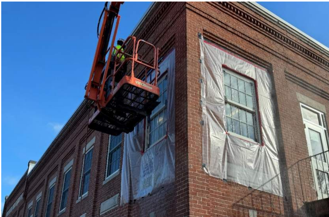
Photo #1 - Building A Pre-Test Window (02/06/24)
