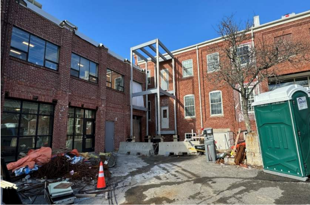
Photo #3 - Building B - Stair Connector in Progress (02/06/24)
