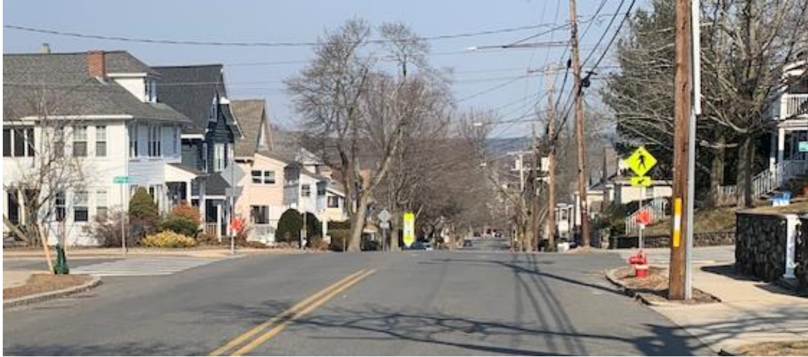
Figure 3: An approach angle headed north where the zebra stripes are less visible, and yield lines are faded.
