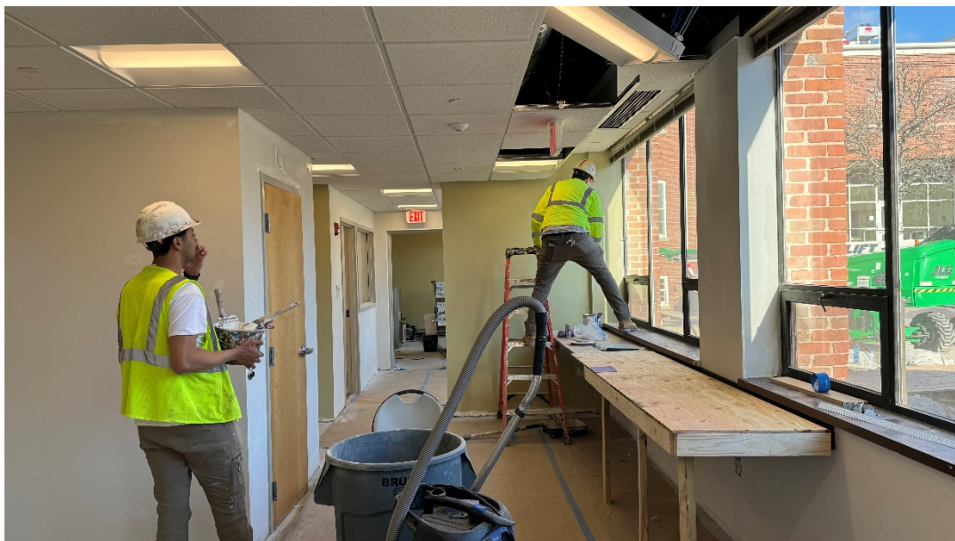
Photo #8 - Building B – Level One Painting in Progress (03/19/24)
