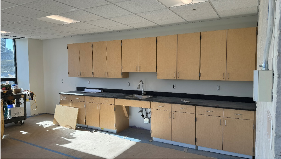
Photo #3 - Building B - Millwork Install in Progress (03/12/24)
