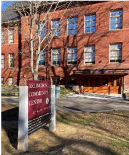
Maple Street main entrance – new sign, entry, canopy
