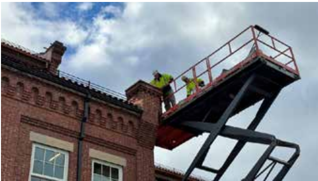
Brickwork and capstone renovations on Building D.
