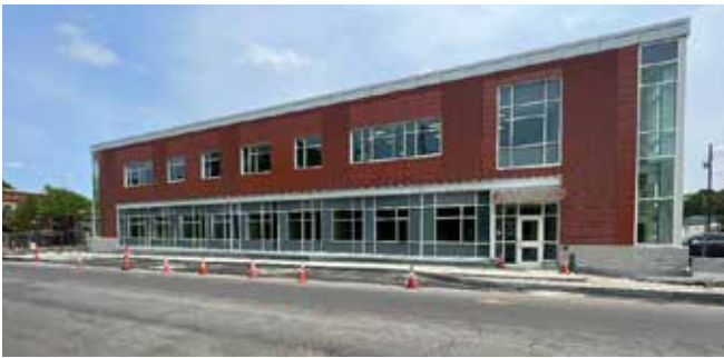
New Building E on Grove Street.
