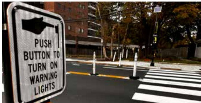
One of many traffic signal upgrades at Chestnut St, includes this solar powered pedestrian crosswalk.
