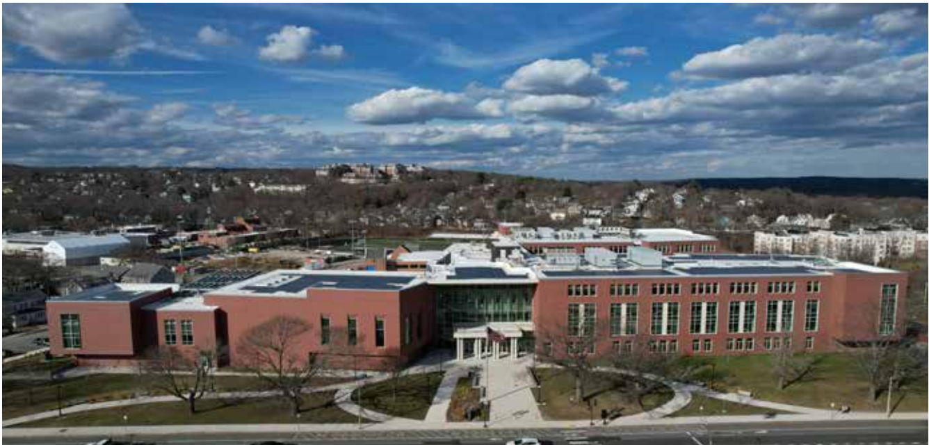
Aerial view of Arlington High School. In 2023, Phase 2 completed and welcomed students and staff to the new Humanities wing, library, and over 40 classrooms.
