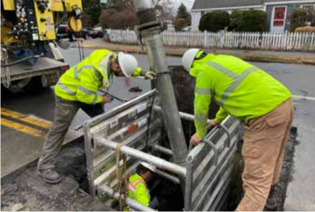
Arlington Water/Sewer Division repairing a water main.
