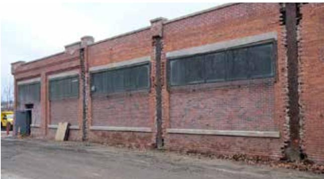
Exposed columns to be repaired and filled on Building D.
