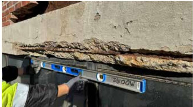
Deteriorating lintels to be repaired or replaced on Building D.
