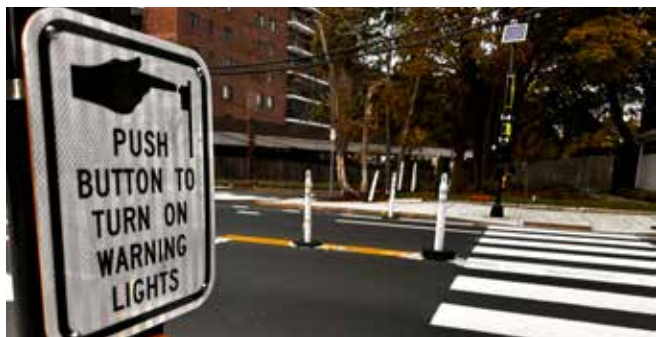
One of many traffic signal upgrades at Chestnut St, includes this solar powered pedestrian crosswalk.
