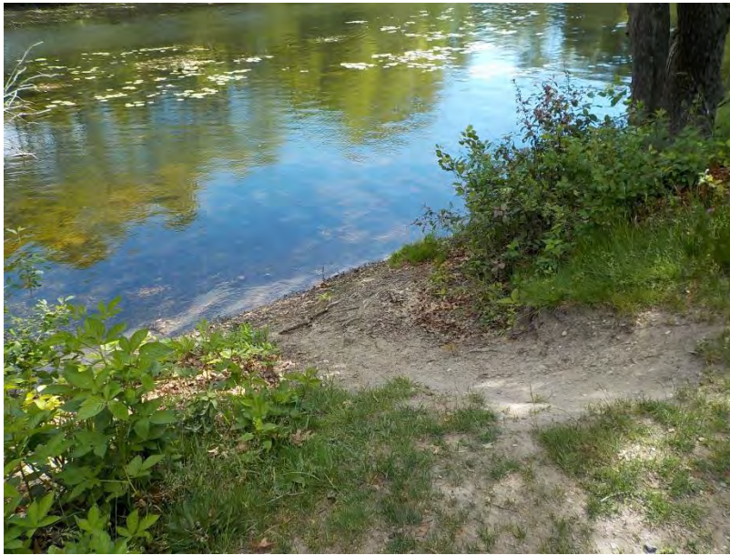
Photo #3: South side of Mystic River, Mystic River Parkway between Location #1 and River Street. Many fishing access points along riverbank are eroded. Note shallow depth of river extending several feet out. (Location #2) (Photo Taken: 06/10/16)
