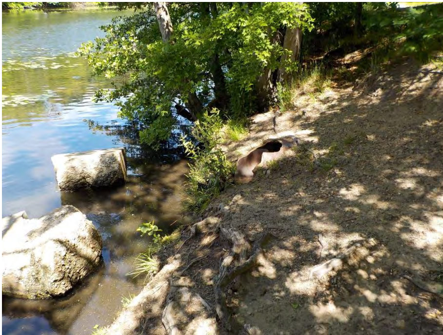
Photo #16: North side of Mystic River, Dugger Park. Eroded banks where humans access the river and pipe discharges. (Location #9) (Photo Taken: 06/10/16)
