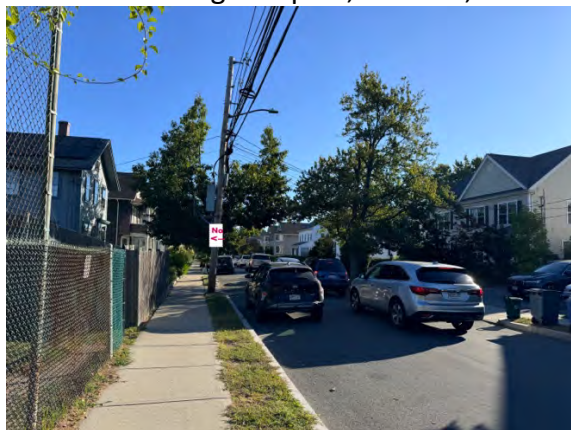
Installation of sign on post, left side, end of park (D1)
