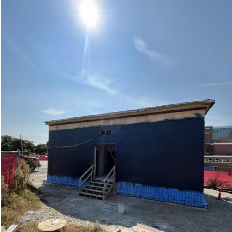
Photograph 3: Toilet Facility Building Exterior
