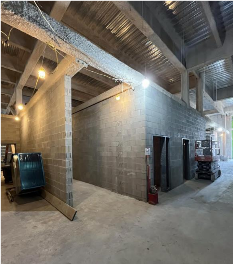
Photograph 1: CMU walls in the locker rooms
