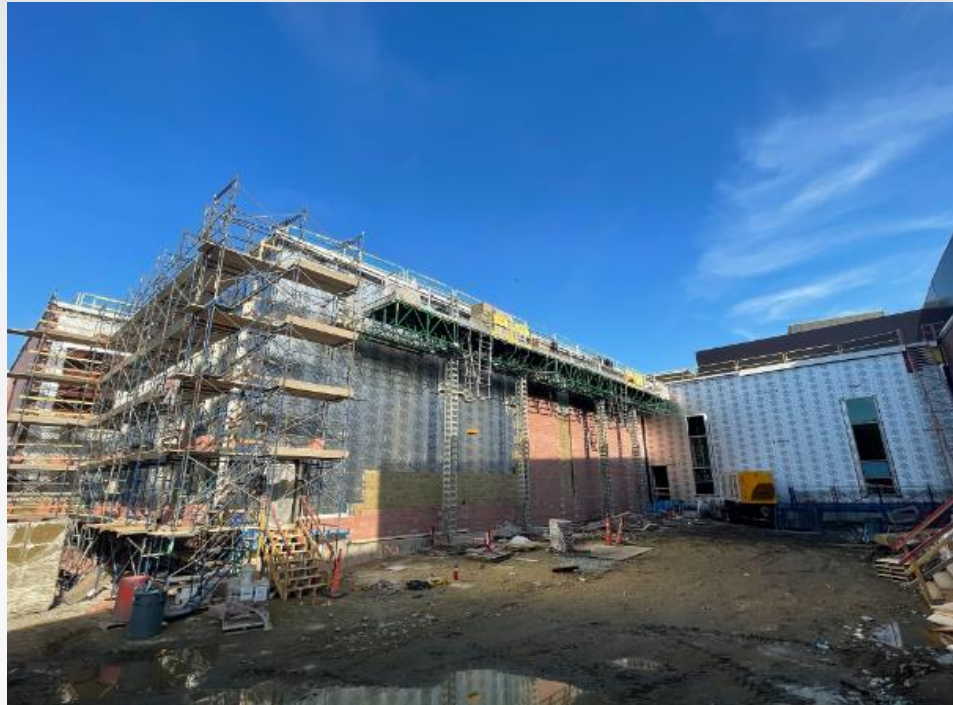
Exterior Building A – South + Blackbox Elevations
