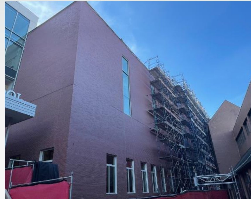
Exterior Building A - North
