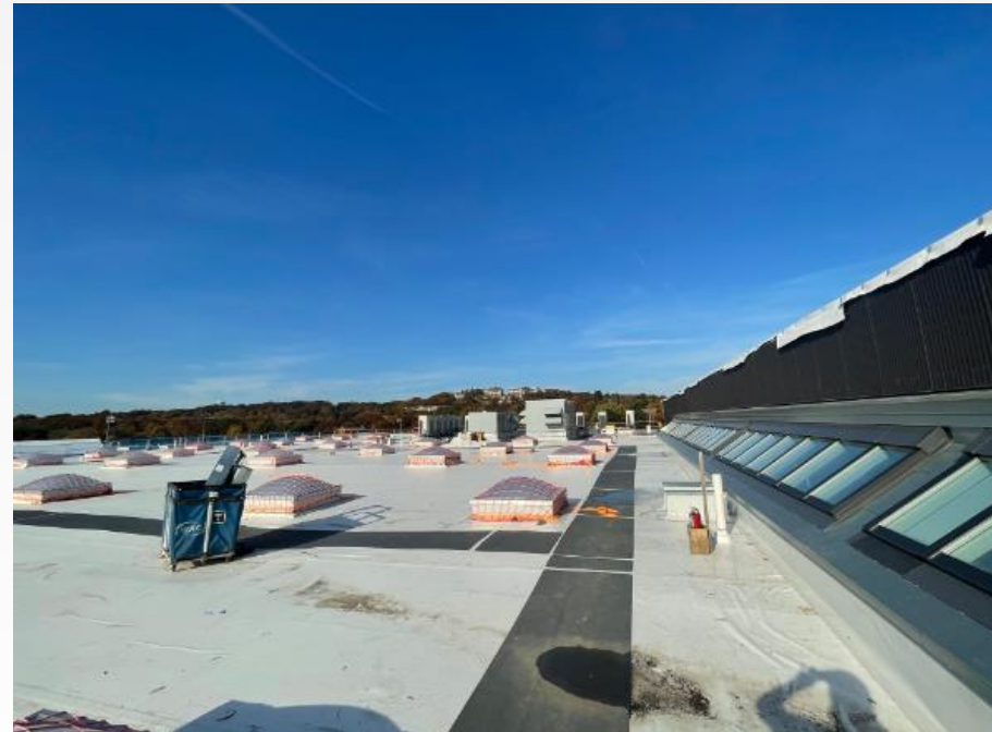
Building A Roof – Metal Panels + Modular Skylight
