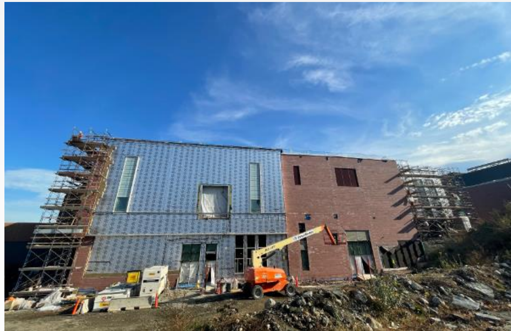
Exterior Building A - West
