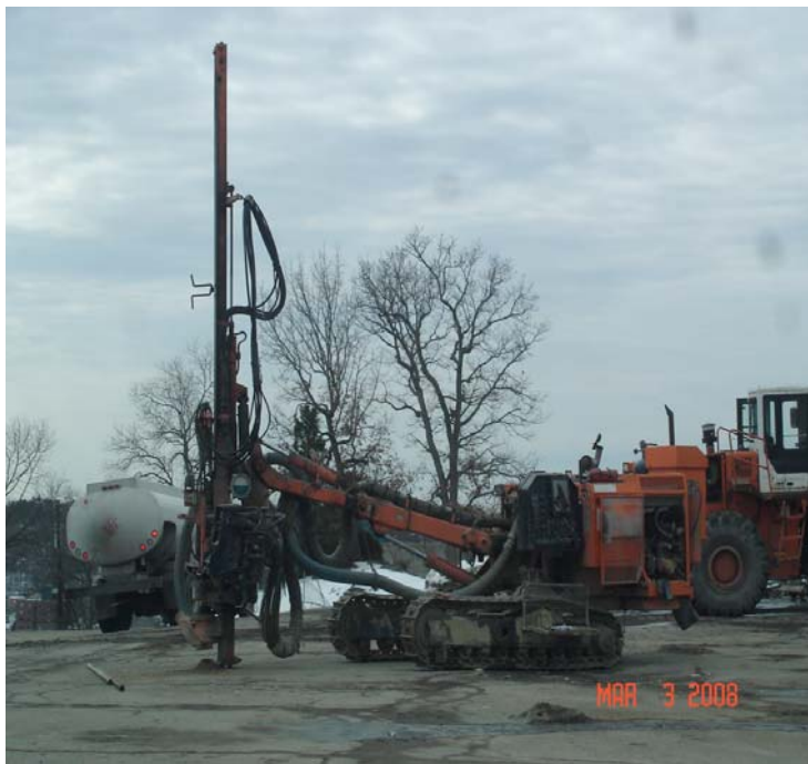
Typical Drill Rig. (Currently on site)
